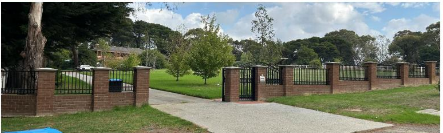
Existing fence along Nortons Lane
