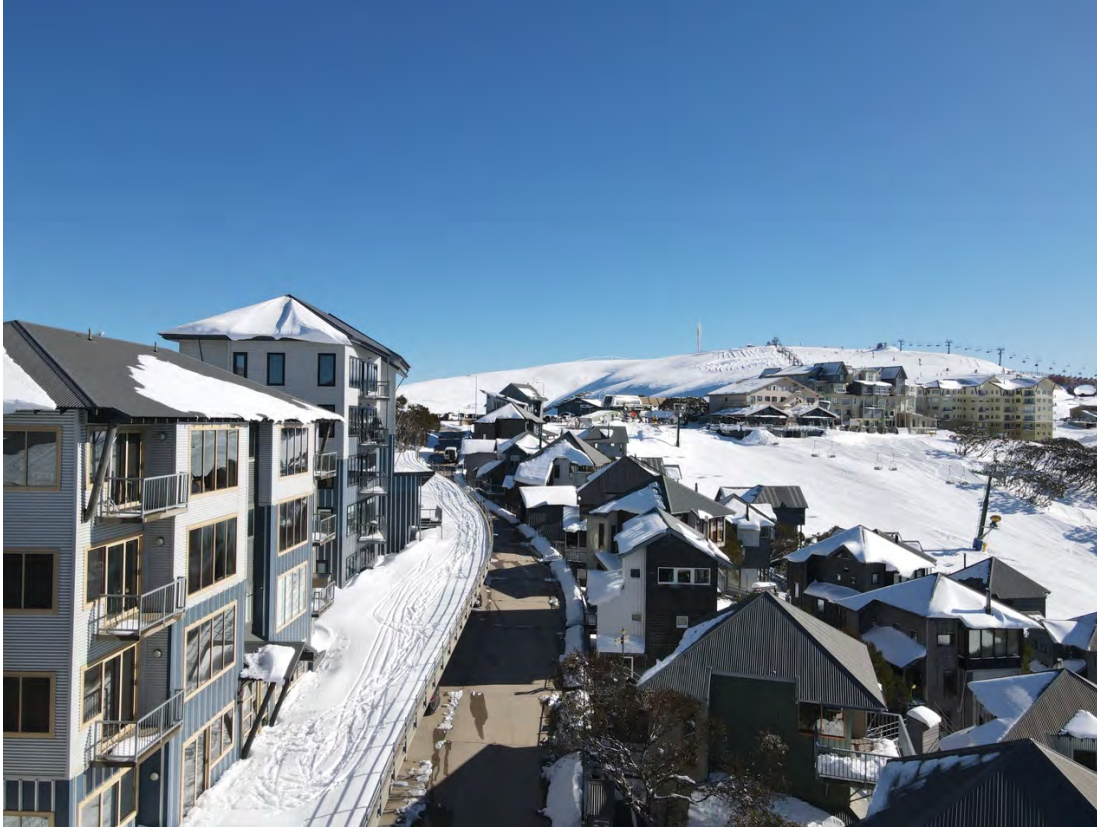
Hot Plate Drive looking north west
