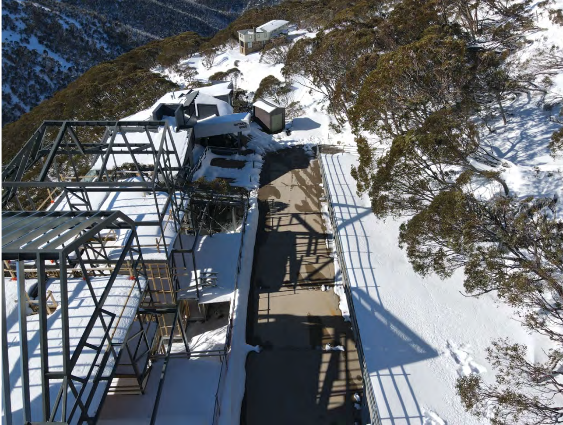
Hot Plate Drive looking south east
