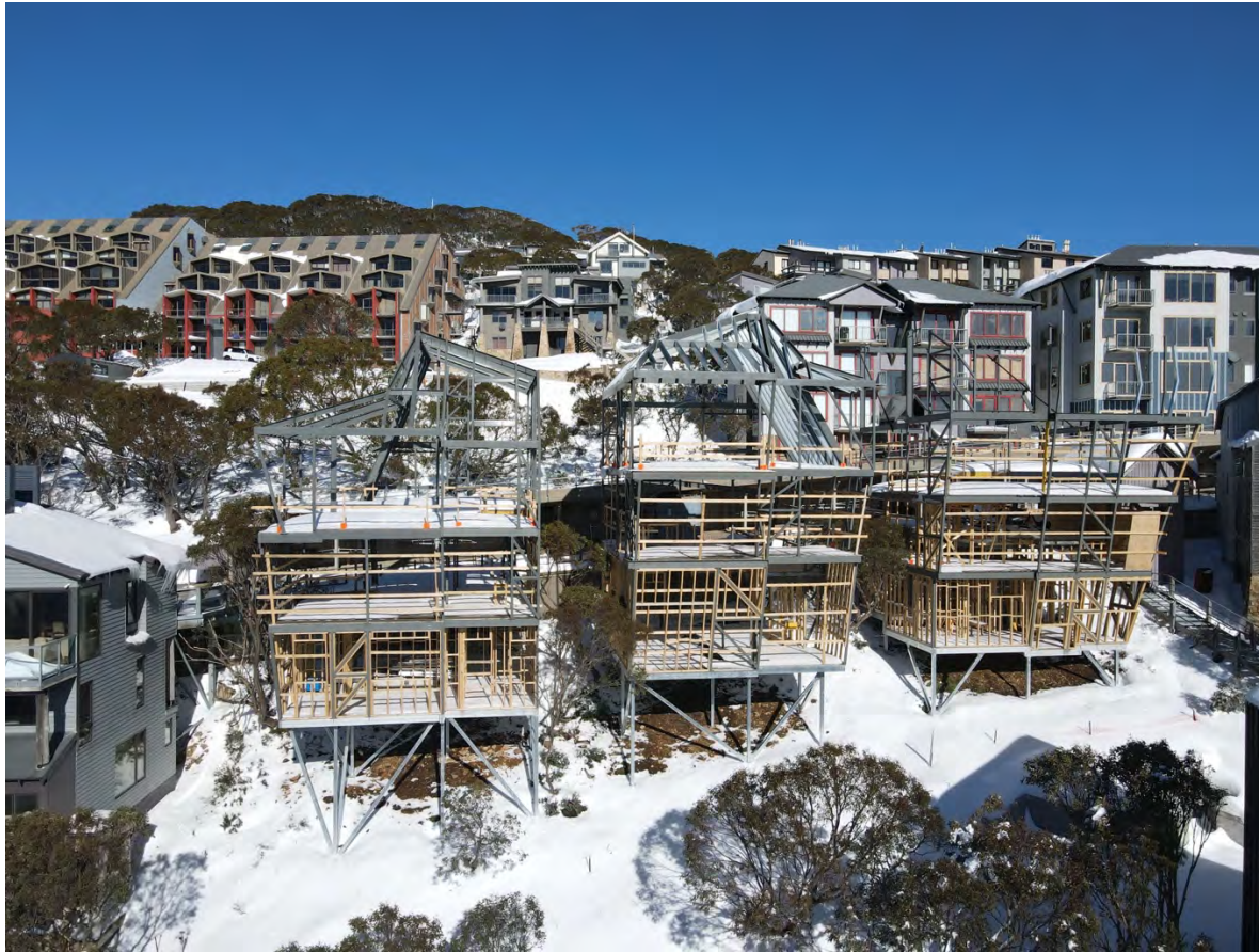
Proposed house site showing south abutting dwellings at under construction
