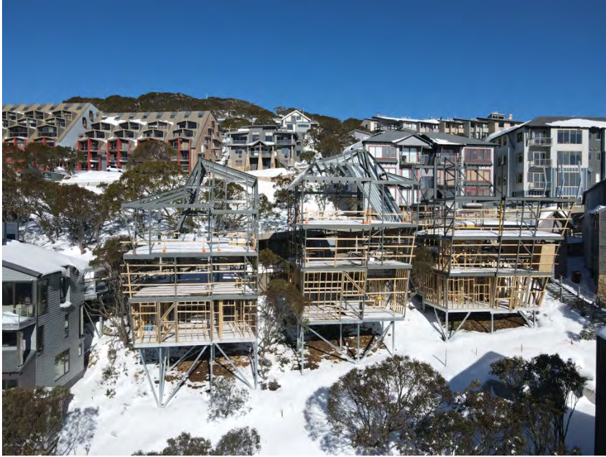
Figure 3.8: Proposed house site showing south abutting dwellings at under construction
