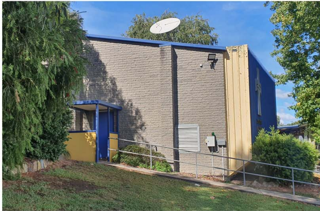
JEN BUILDING - LECTURE THEATRE. EXISTING CONDITIONS. RE-CLADDING AND PAINTING WORKS.
