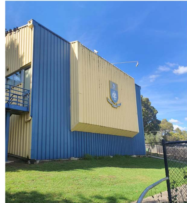
CAM BUILDING - DANCE STUDIO EXISTING CONDITIONS. RE-CLADDING AND PAINTING WORKS.
