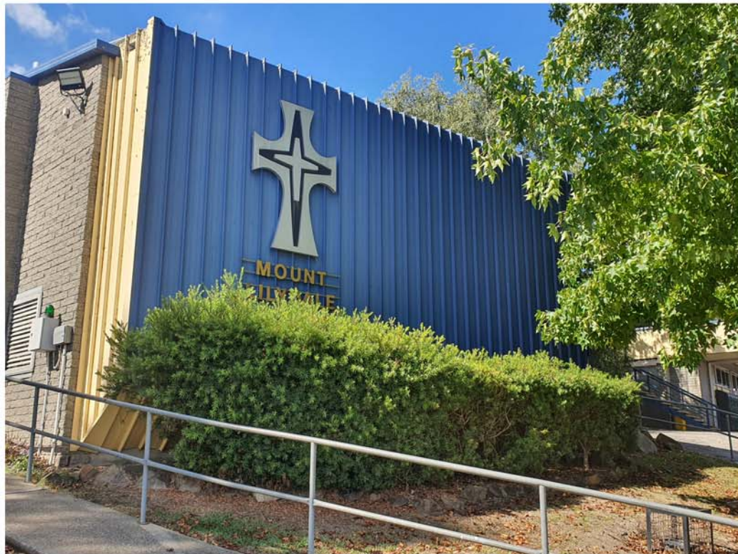
JEN BUILDING - LECTURE THEATRE. EXISTING CONDITIONS. RE-CLADDING AND PAINTING WORKS.
