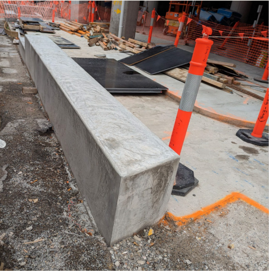
Off Form Concrete Wall | 25mm Radius to Top Edge
