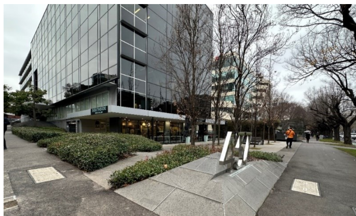
Figure 4: View of subject site from the corner of St Kilda Road and Slater Street
