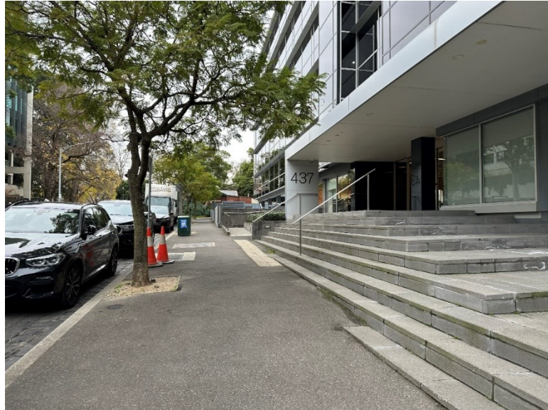
Figure 7: View east along the subject site's frontage to Slater Street to lobby entrance
