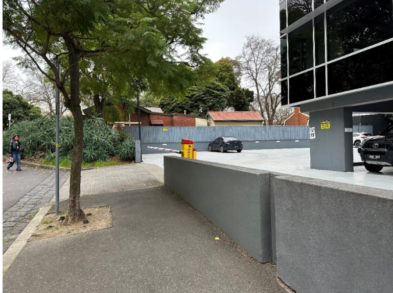
Figure 9: View east to rear vehicle crossover to the rear along Slater Street and caretaker cottages behind
