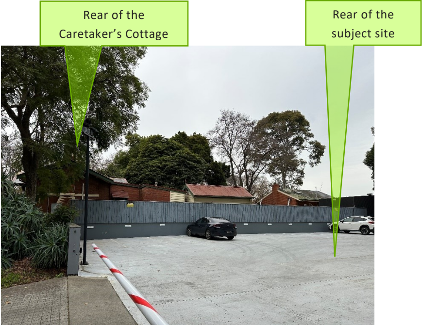
Figure 17: View from the rear crossover along Slater Street to the rear of the heritage significant Fawkner Park Caretaker's Cottage and depot
