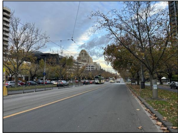
Figure 5: St Kilda Rd Central Carriageway – View South
