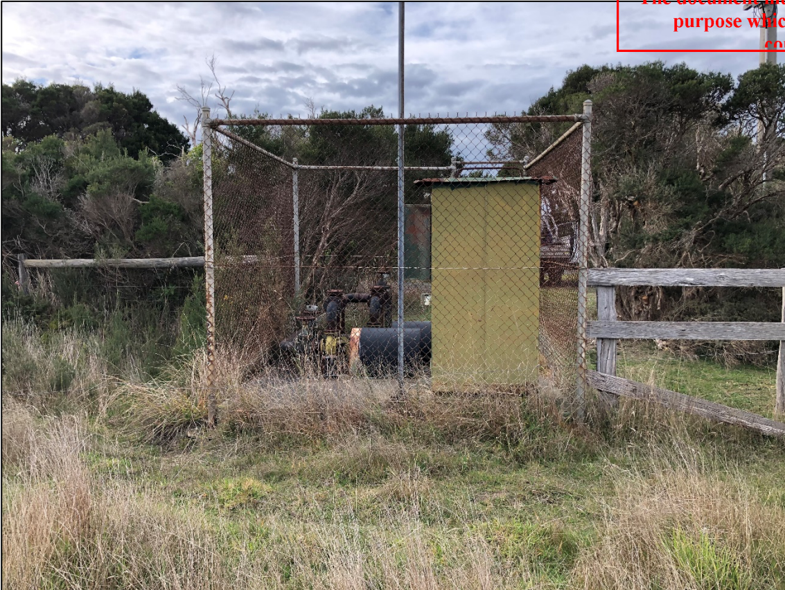
Figure 6: Existing pumping station to be retained.
