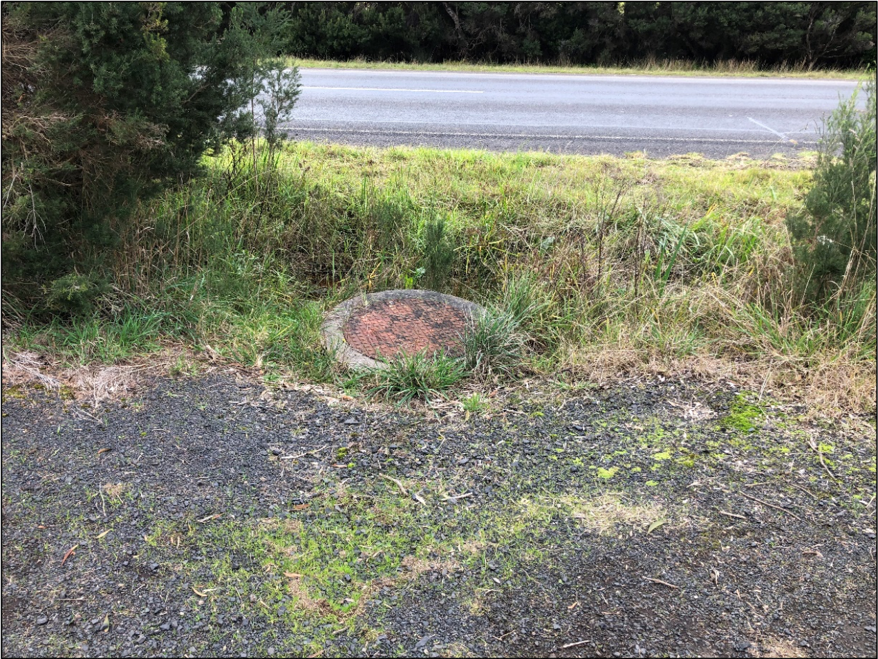
Figure 7: Sewer access pit present in AC1 to be avoided.
