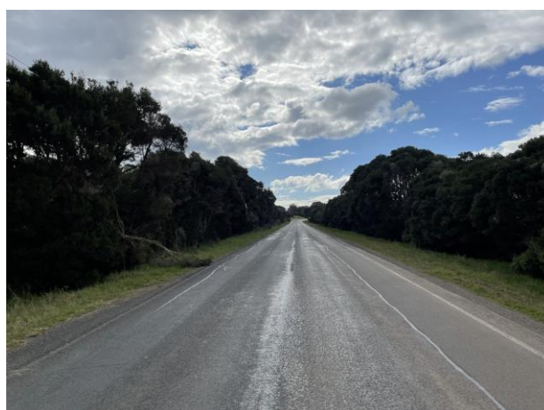
Photograph 8 – View north along Gap Road
