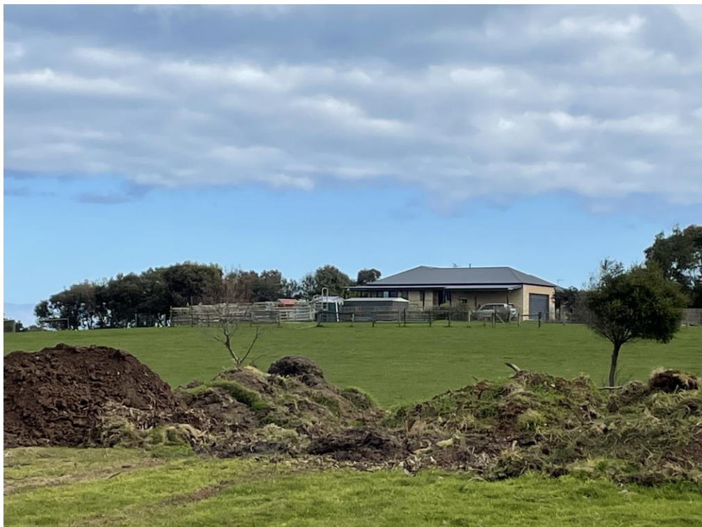
Photograph 7 – View west from Ventnor Road to the nearest dwelling
