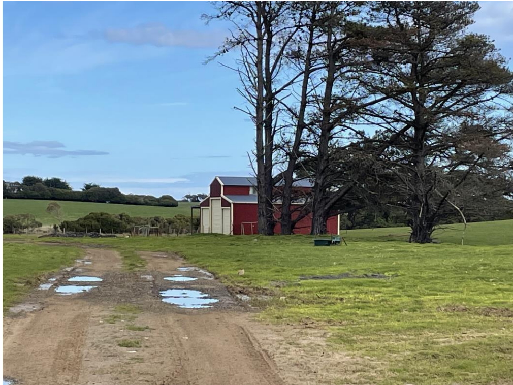
Photograph 6 – View south from Ventnor Road to the nearest building (barn)
