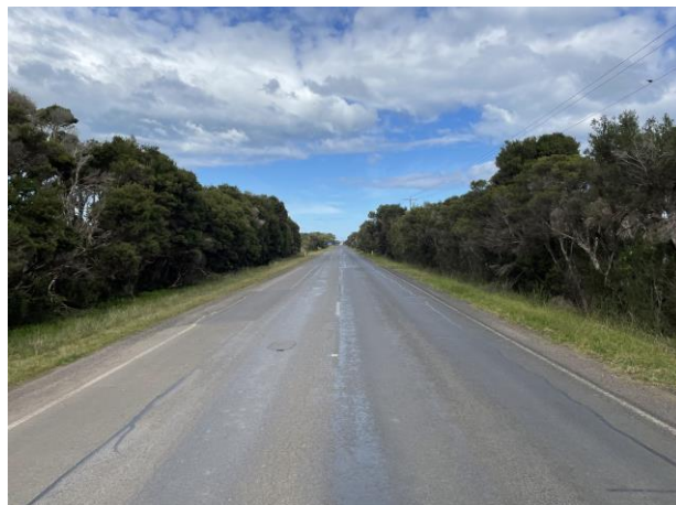
Photograph 9 – View south along Gap Road
