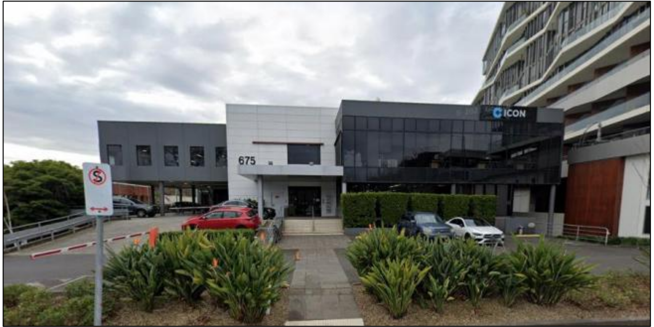
Figure 9: Victoria Street frontage (Source: Application)
