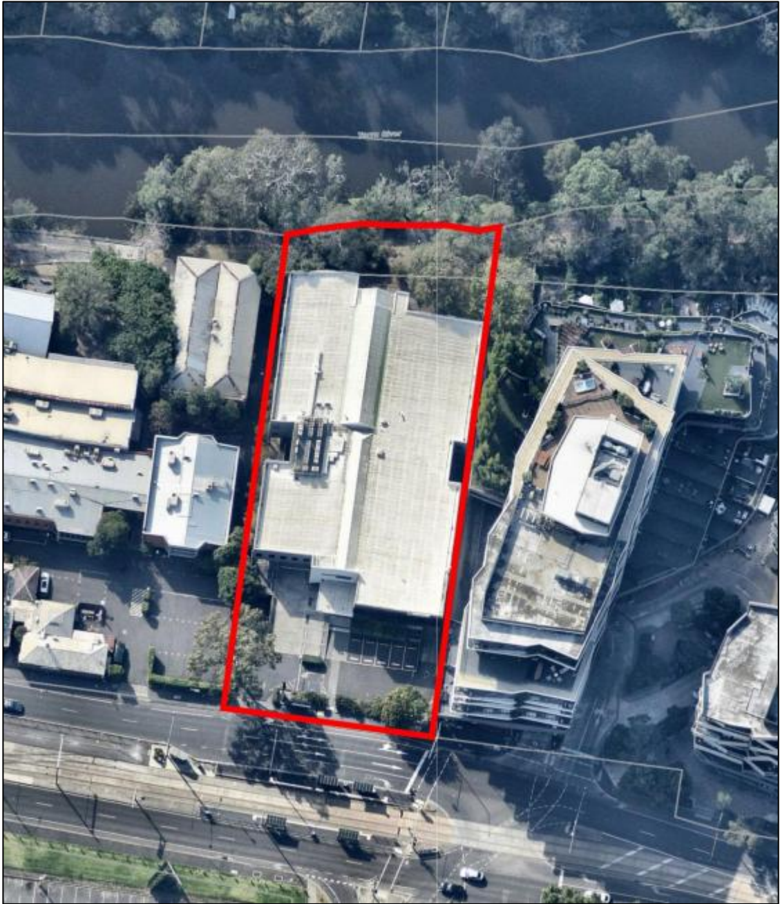
Figure 8: Subject site (Source: Application)
