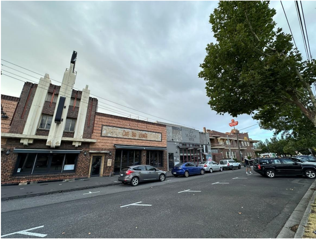
Figure 15: Subject site as viewed from Queens Parade (looking west)
