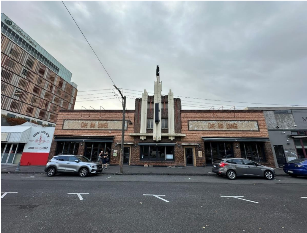
Figure 13: Subject Site as viewed from Queens Parade (north-west elevation)
