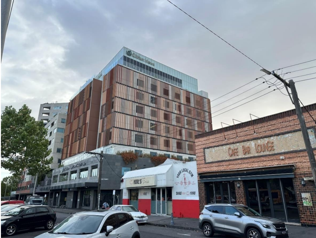
Figure 14: Subject site as viewed from Queens Parade (looking east)
