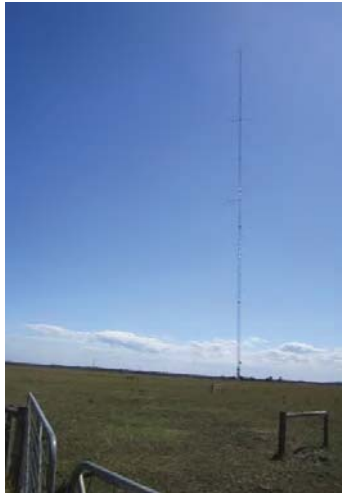
Existing 80m Met Mast (close up)
