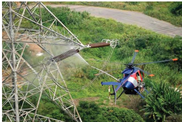
Washing insulators using a MD 500 helicopter.
