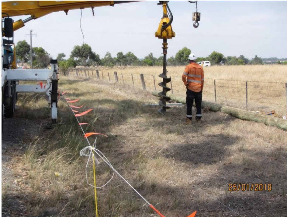
Figure 3: Example of a hole being augured via arm from truck (note in this example the roadside vegetation was deemed to be native in places and fencing was set up to keep the truck from the shoulder)
