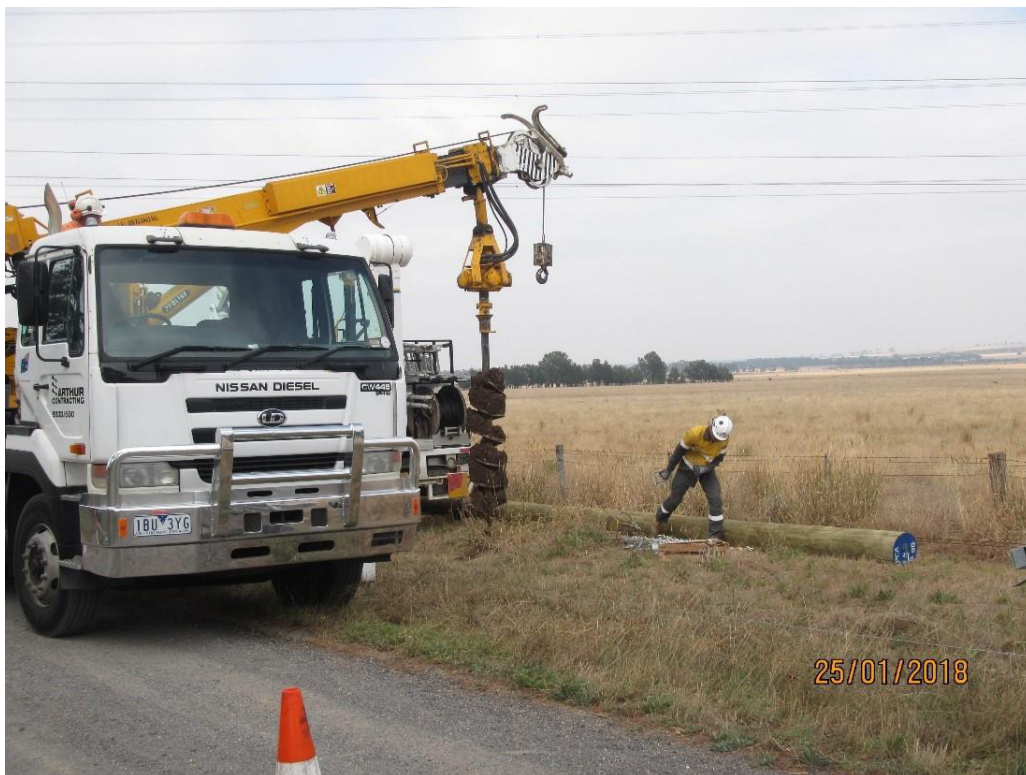
Figure 2: Example of a hole being augured via arm from truck (note in this example the roadside vegetation was deemed to be non-native, hence the truck is parking slightly on the verge and the other truck in the background)
