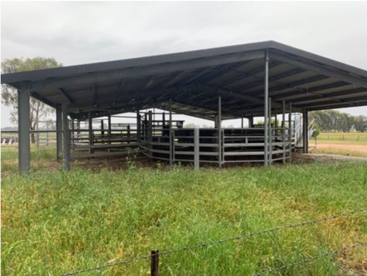
Figure 2-3: Current covered stockyards on property in December 2022
