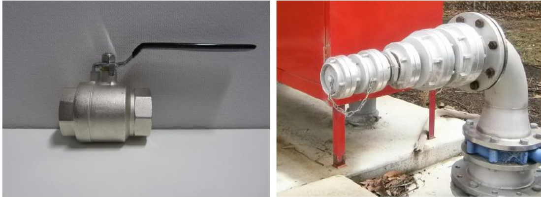
Figure 1 The 150mm full bore isolation valve (shown on the left) and the 125mm x 90mm, 75mm and 65mm Storz tree adapters (shown on the right)
