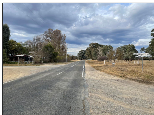
Figure 6 Wangaratta-Whitfield Road facing south
