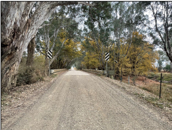
Figure 11 Docker–Carboor Road Bridge 4
