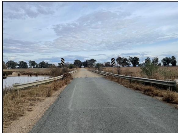
Figure 12 Docker–Carboor Road Bridge 5
