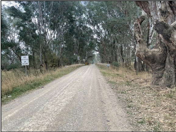
Figure 9 Docker–Carboor Road Bridge 1
