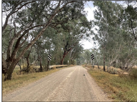
Figure 10 Docker–Carboor Road Bridges 2 and 3
