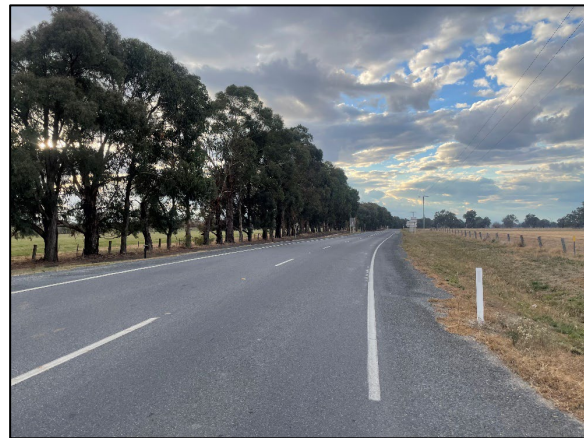
Figure 4 Snow Road facing east
