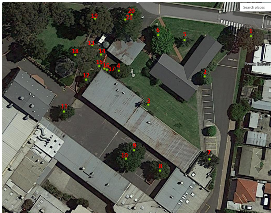
Figure 1. Overhead Site Image existing buildings.
