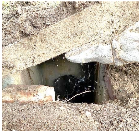
Image 50: Stormwater pit & pipe 2.4m from boundary adjacent Tree 119.
