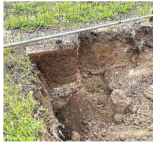
Image 49: Brick wall footing Hawthorn Rd boundary.
