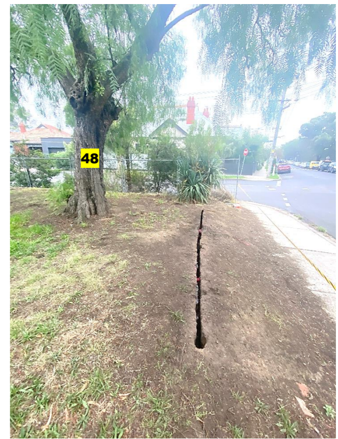
Image 12: Tree 48 two rots located 20mm, 35mm.
