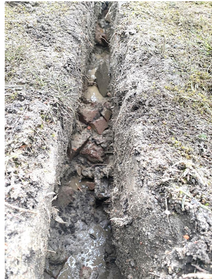
Image 7: Bricks located in trench adjacent to Trees 19, 21, 32, 33.
