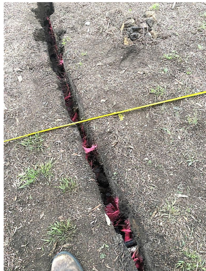
Image 6: Typical of the roots located adjacent to Trees 19, 21, 32, 33.
