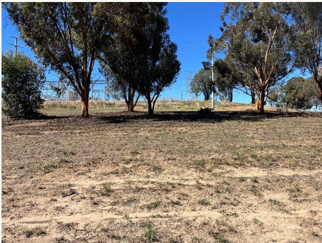
Plate 10: Eastern extent of the road reserve and 576 Winton-Glenrowan Road, showing the Glenrowan Terminal Station infrastructure
