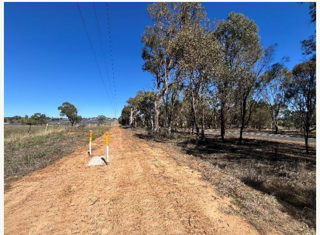
Plate 11: Mid-section of the road reserve, showing the service road with utilities
