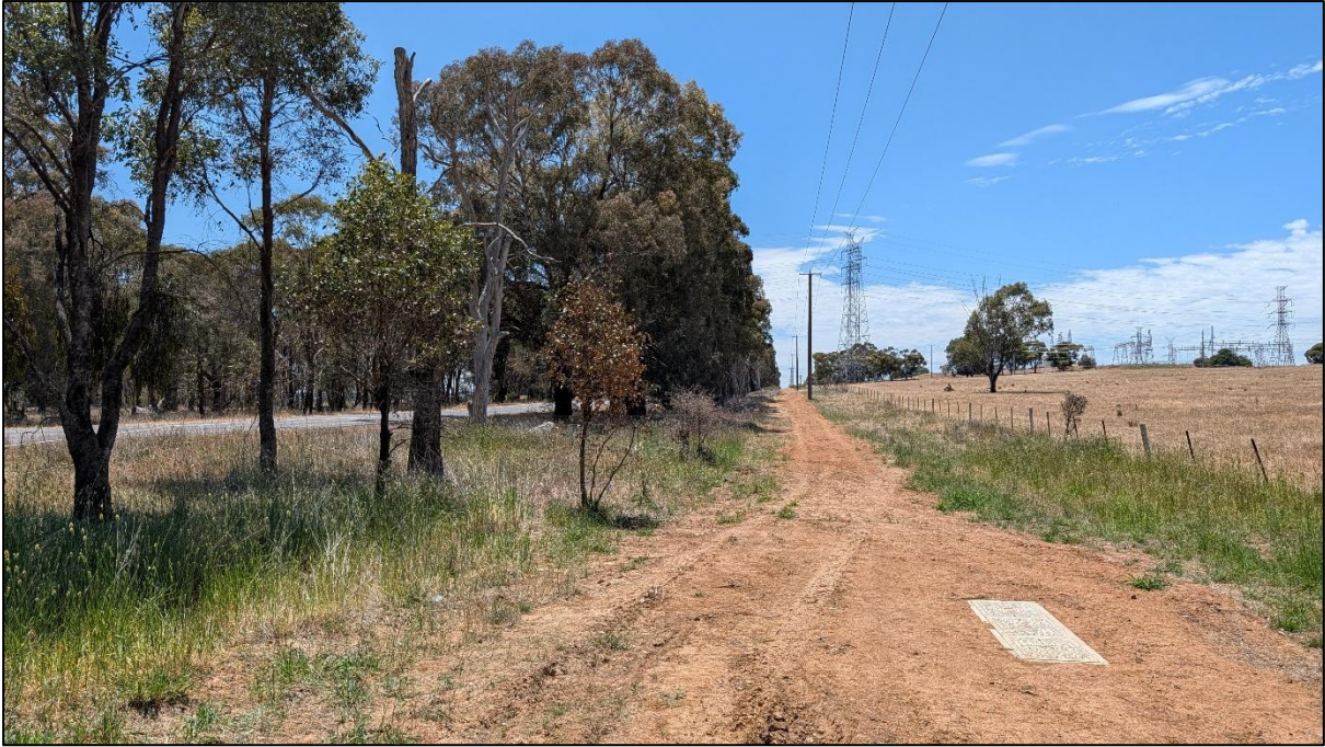
Figure 6: Recent telecommunications work in road reserve, patch 1a on the left (November 2025)
