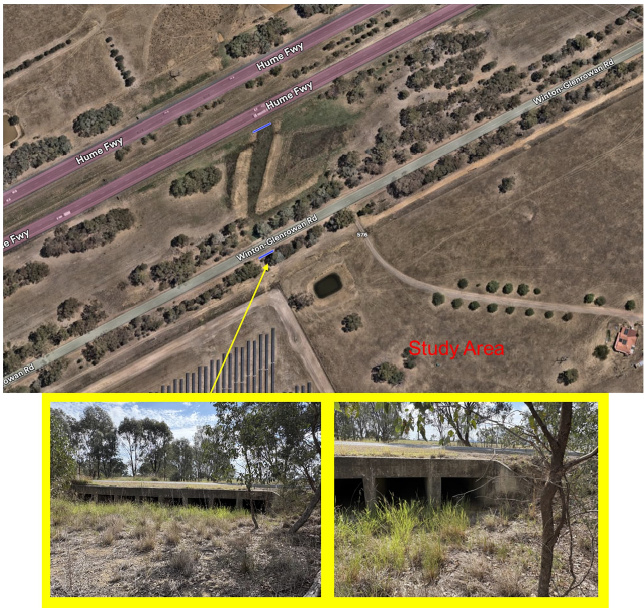
Figure 5: Location and photos of culverts
