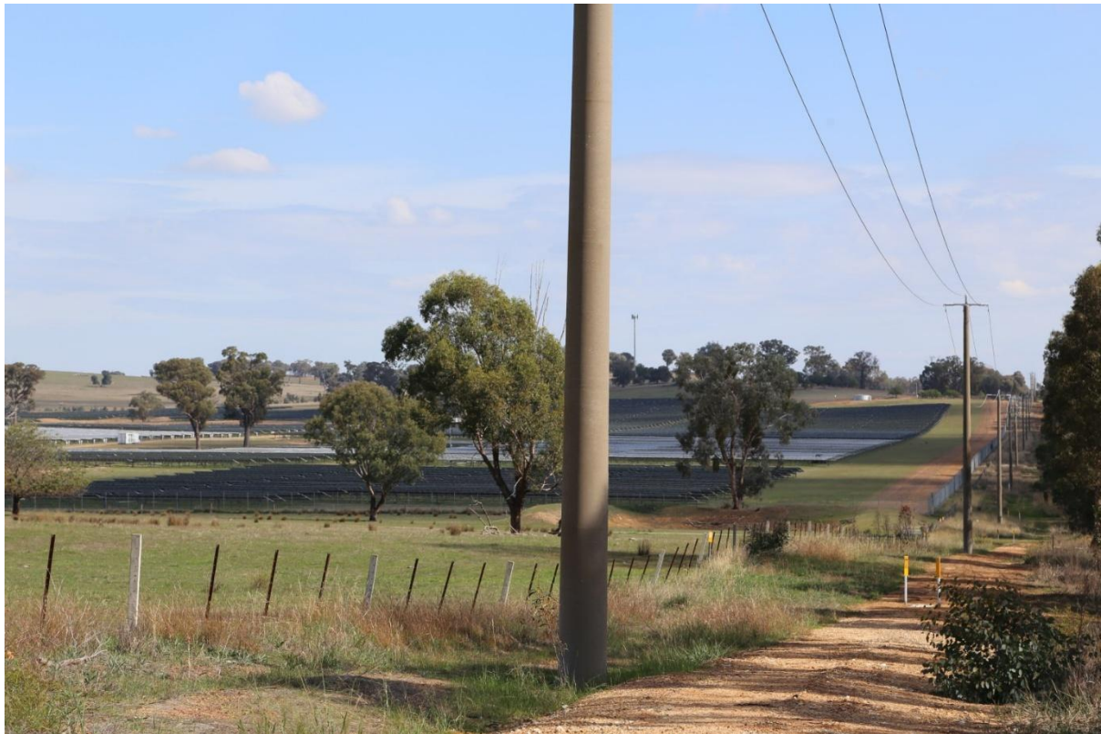
Figure 16 - Winton Solar Farm as viewed from the southern verge Winton-Glenrowan Road, near the Project area.
