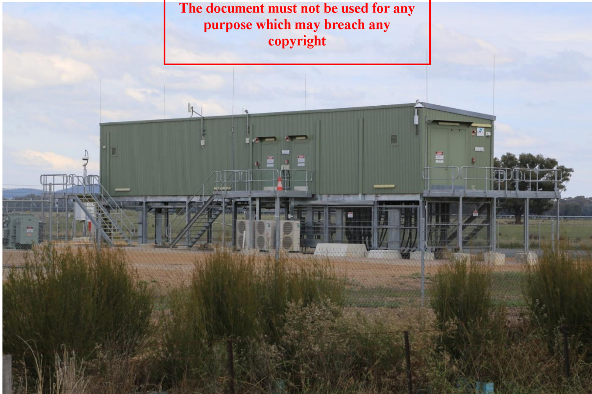
Figure 74 – HV switchroom at Glenrowan West Solar Farm clad in a recessive natural colour.
