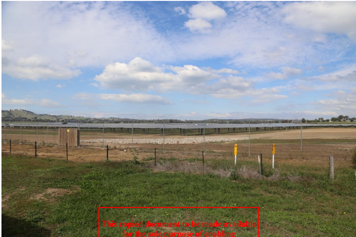
Figure 17 - Glenrowan West Solar Farm as viewed from Winton-Glenrowan Road.
