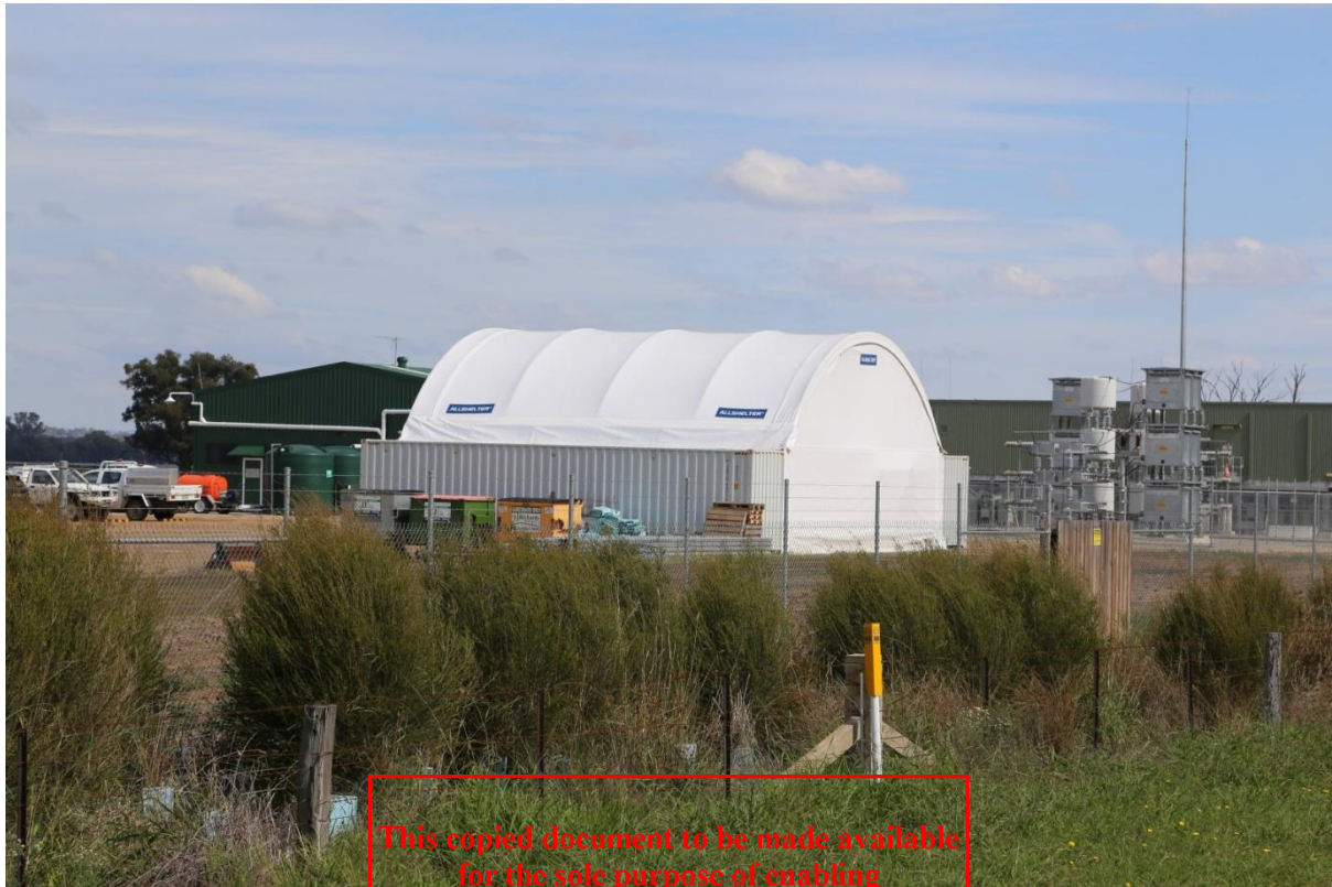
Figure 75 – High contrasting colours, such as at the storage and maintenance area at Glenrowan West Solar Farm, should be avoided where possible.
