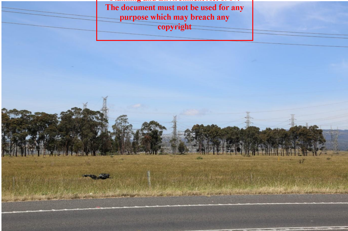
Figure 76 - Example of canopy vegetation providing visual integration of substation infrastructure.
