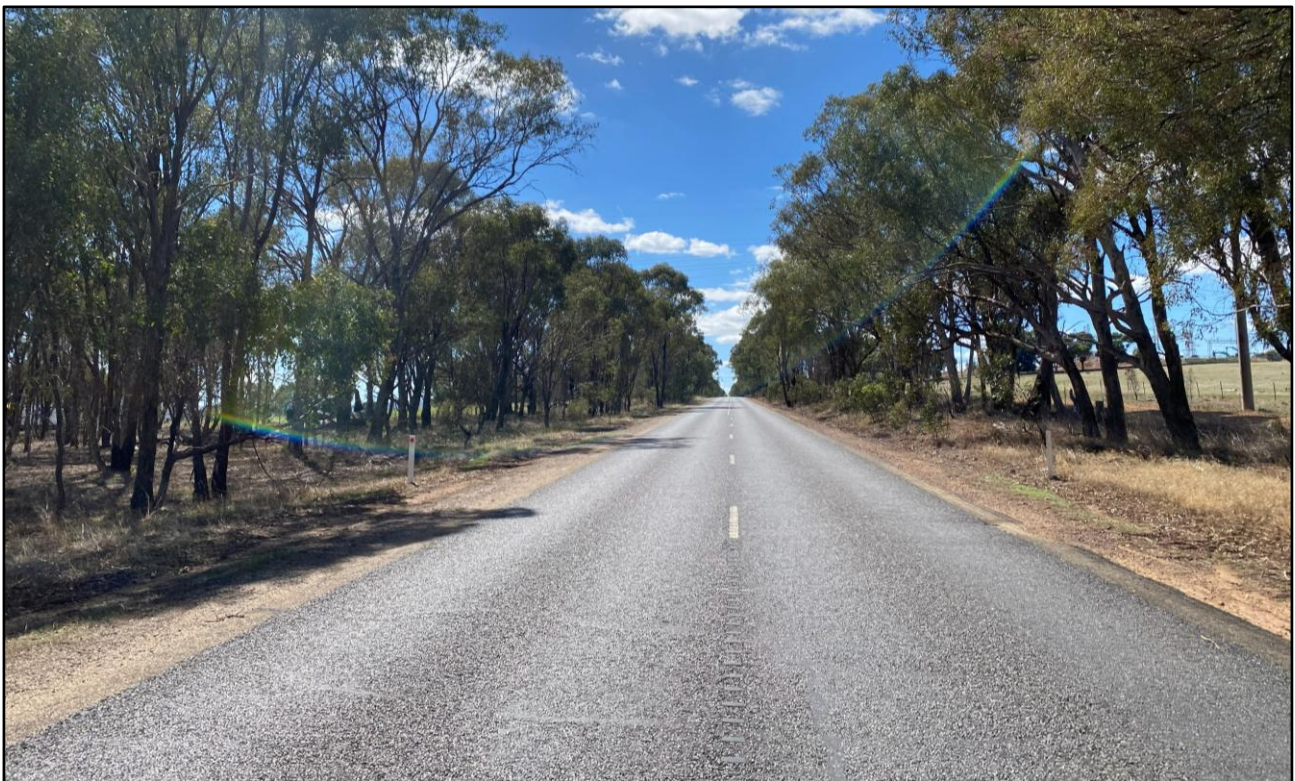
Figure 3 Winton-Glenrowan Road, looking east adjacent to the subject site
