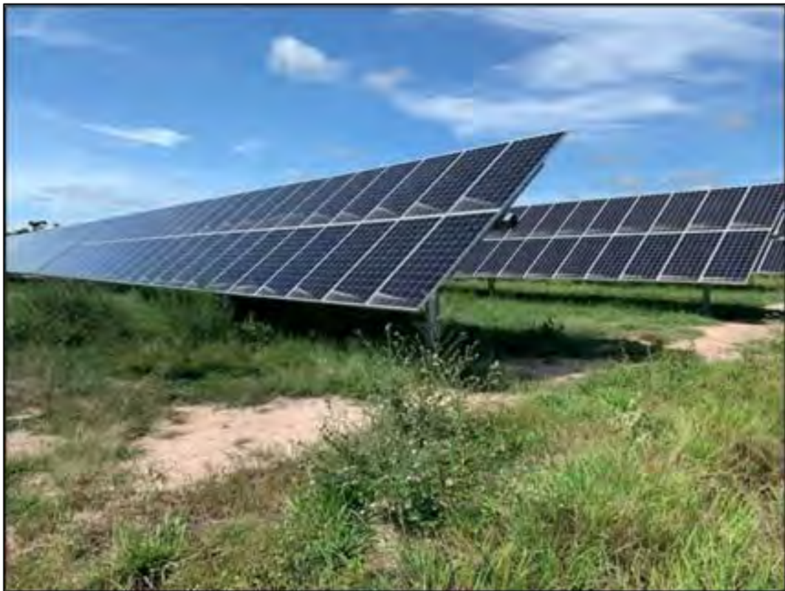
Figure 5. Real-life example of vegetation growth below a single axis tracker PV system.
