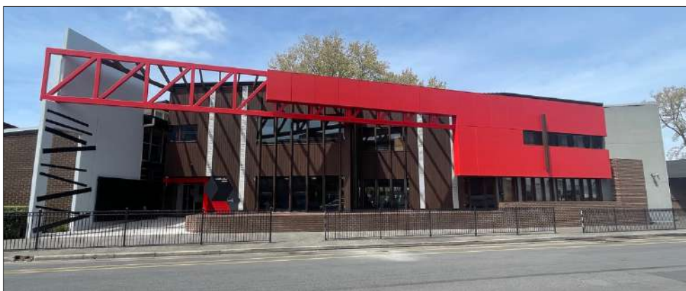
Figure 23 Ballarat Clarendon College's Year 7/8/9 building - also located in the West Ballarat Precinct.
