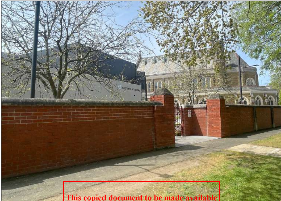
Figure 14 View from Sturt Street showing the Mary's Mount Centre (left) and Chapel (right). The historic red-brick boundary wall is visible in the foreground.
