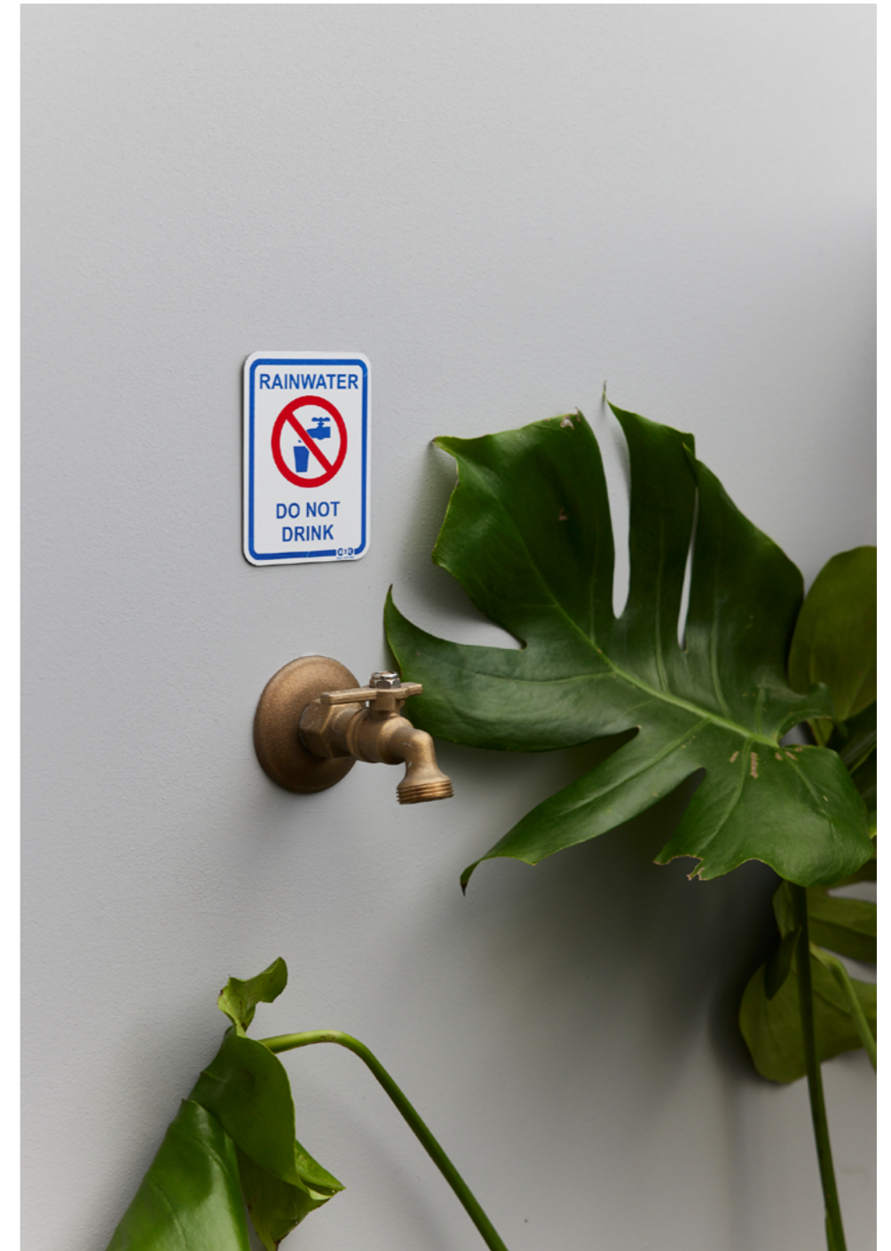
Rainwater connections to balcony taps at Ferrars & York. Photography by Kim Landy.
