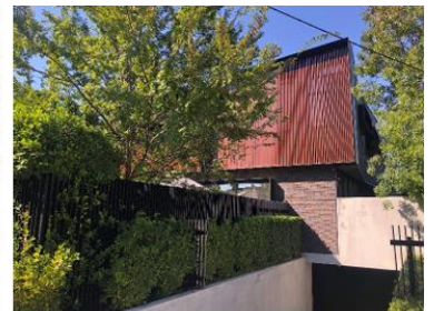
Figure 16 – The contemporary, flat roofed townhouse complex at 8 Manningtree.
