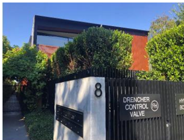
Figure 15 – The contemporary, flat roofed townhouse complex at 8 Manningtree.
