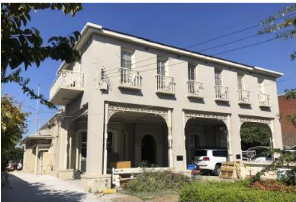
Picture 1 Subject site (existing Manor House), looking south Source: Site, 18 March 2024
