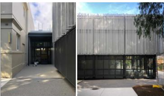
Picture 2 Single storey link Picture 3 New multi-purpose centre Source: Smith + Tracey Architects, on site 5 June 2024
