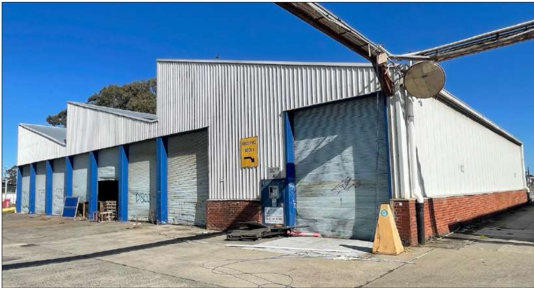
Figure 51 The east elevation of building 7.
