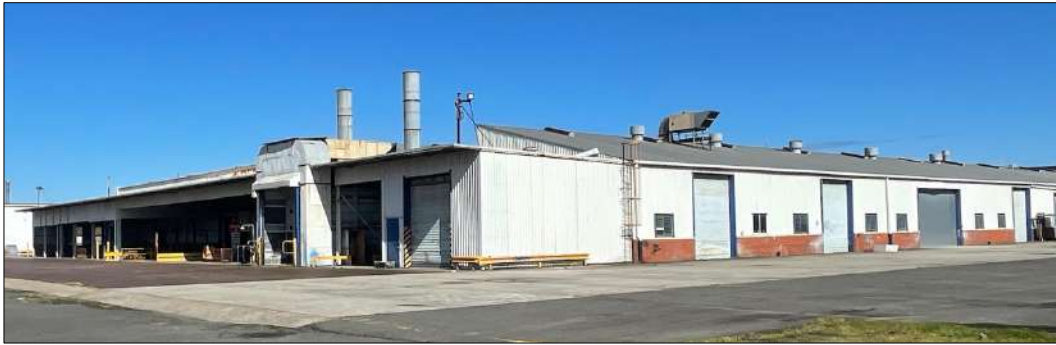
Figure 46 The 1965 additions to the factory viewed from the north-east.
