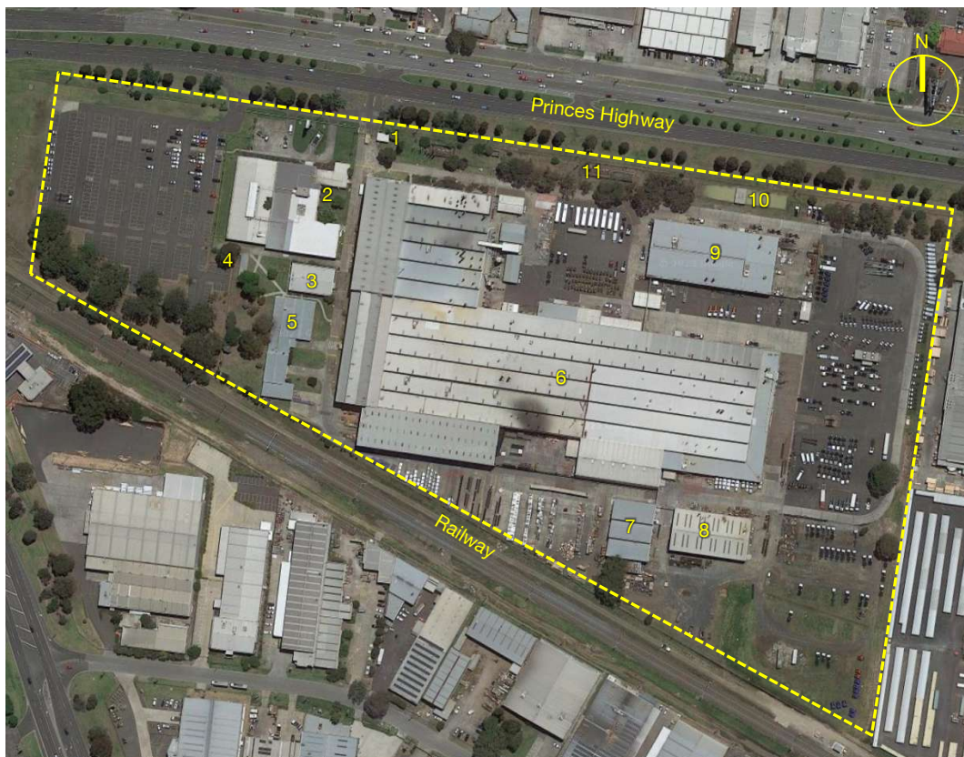
Figure 22 Aerial photograph of the former International Harvester factory site. Numbered buildings are described below.
