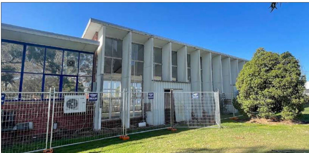
Figure 35 Vertical sun baffles to the west elevation of the amenities block.
