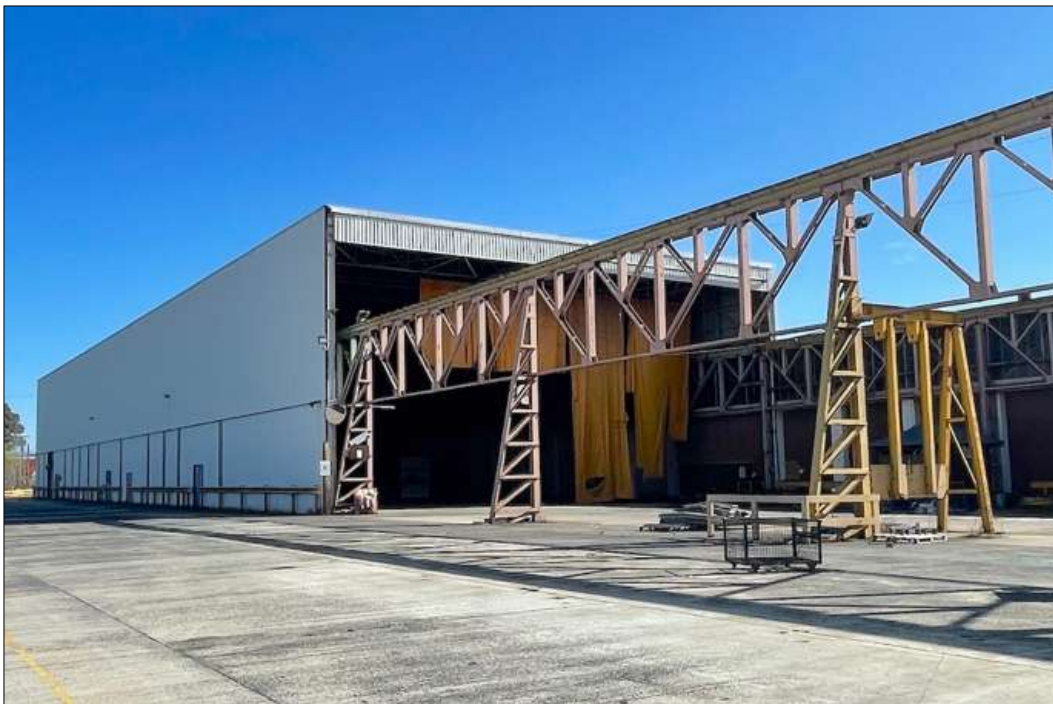
Figure 43 The c1968-72 addition to the south of the crane bay, and original steel crane gantry.
