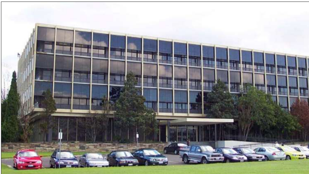
Figure 62 Ford Motor Company administration building, Broadmeadows.
