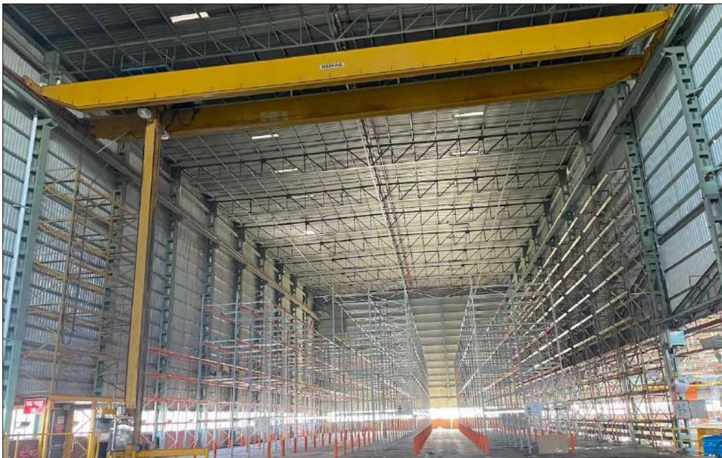
Figure 45 The interior of the c1968-72 addition to the north of the crane bay.
