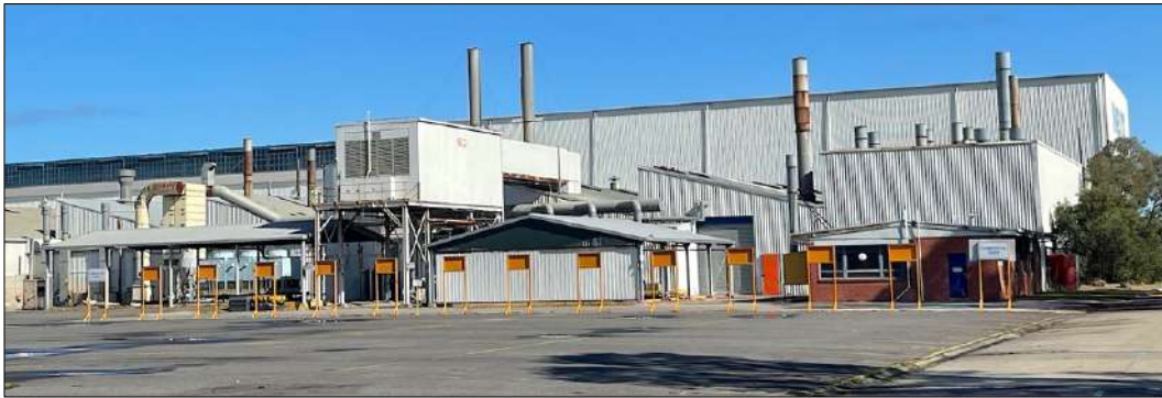
Figure 47 Various ancillary structures on the east side of the factory, typically dating from the 1980s and 1990s.
