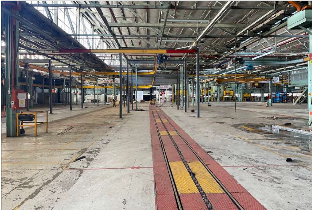
Figure 49 Assembly line interior showing chain conveyor set into the floor.
