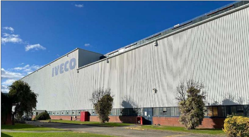
Figure 42 The west elevation of the crane bay. The c1968-72 addition is visible to the left.
