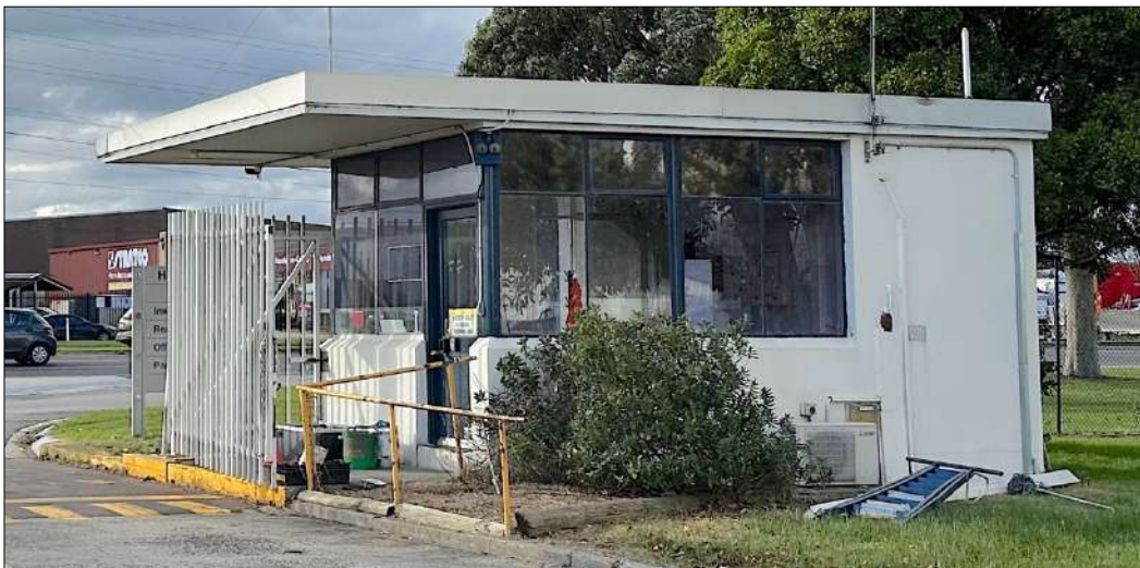
Figure 24 The gatehouse viewed from the south.
