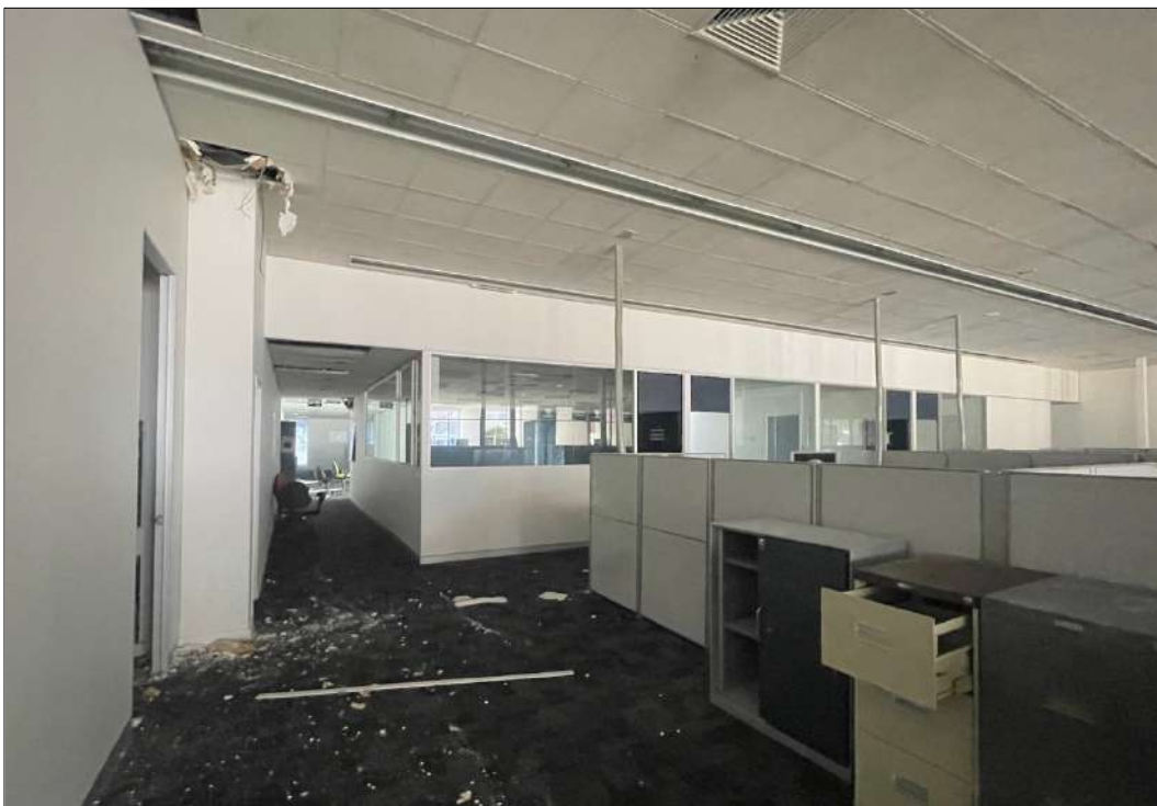
Figure 31 Typical interior in the administration building.
