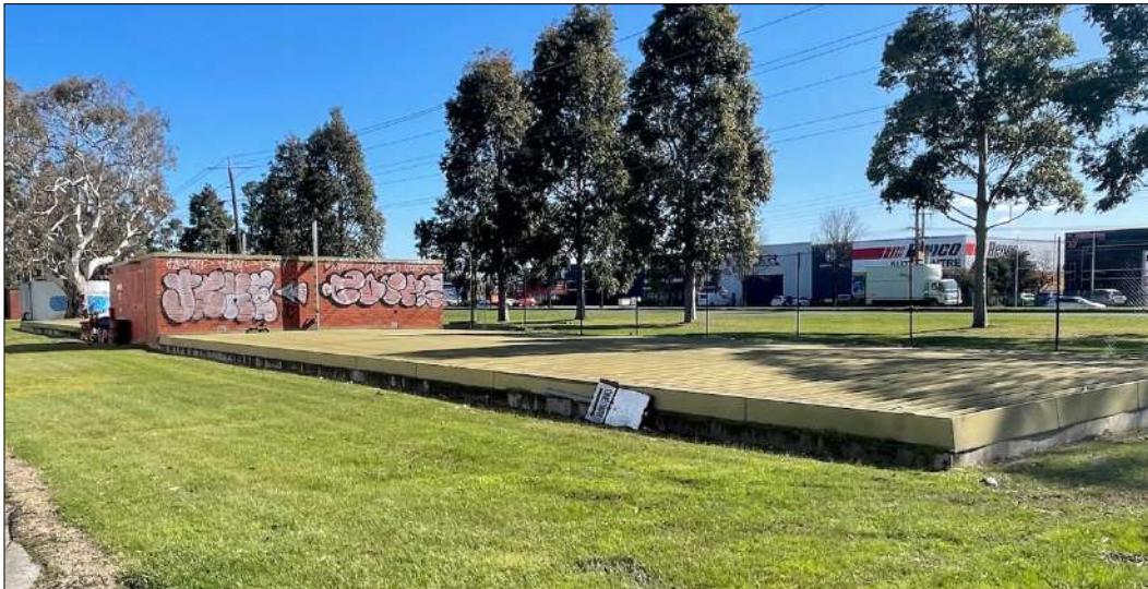
Figure 55 Water tanks and pump house.
