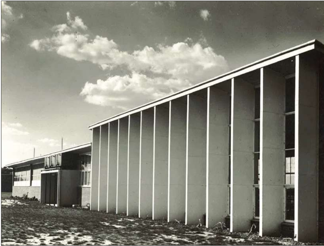
Figure 11 The west elevation of the amenities block showing asbestos cement clad sun baffles, c1953. Source: Hassell
