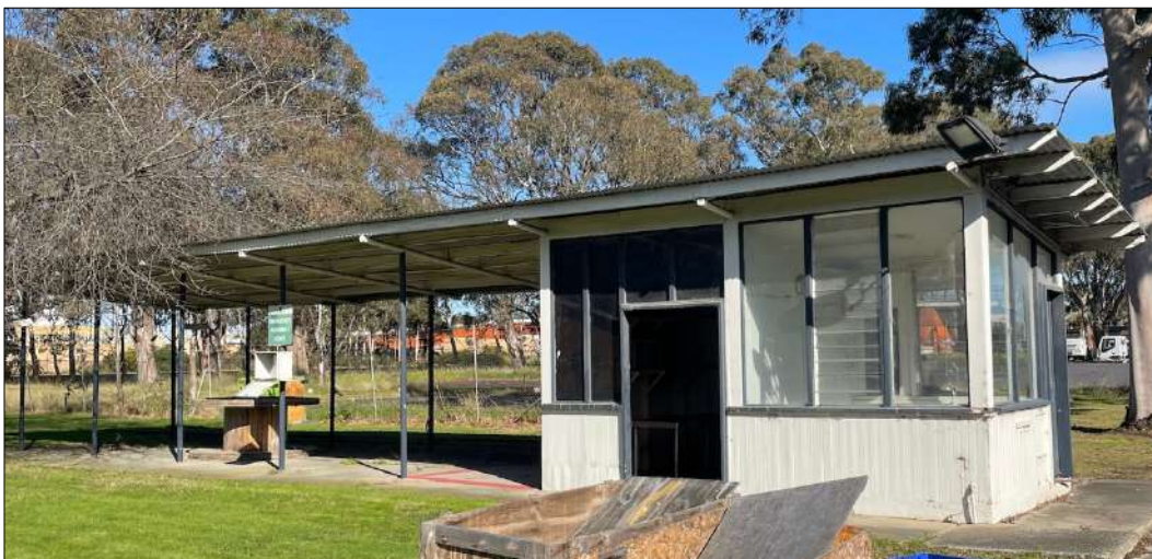
Figure 33 The bicycle shed.
