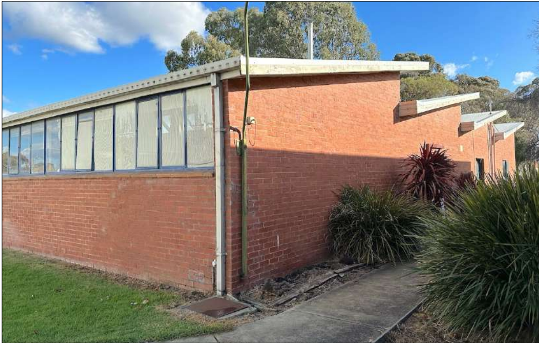
Figure 36 The sawtooth roofs at the northern end of the amenities block.
