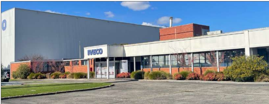
Figure 25 The Princes Highway (north) façade.
