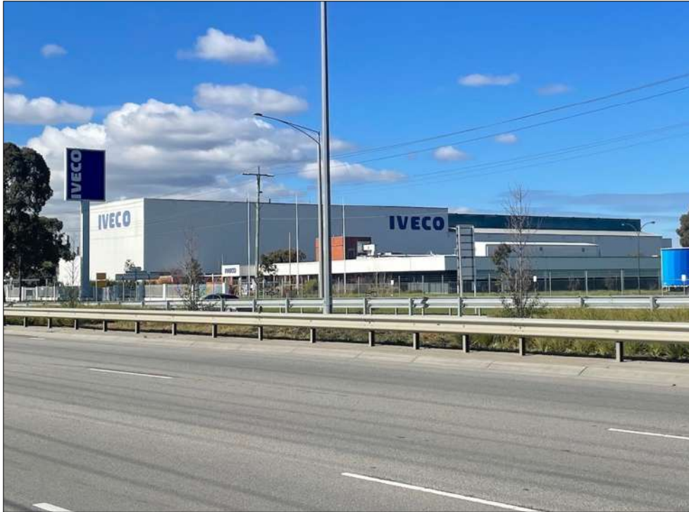
Figure 10 The former International Harvester factory viewed from the west on the Princes Highway.
