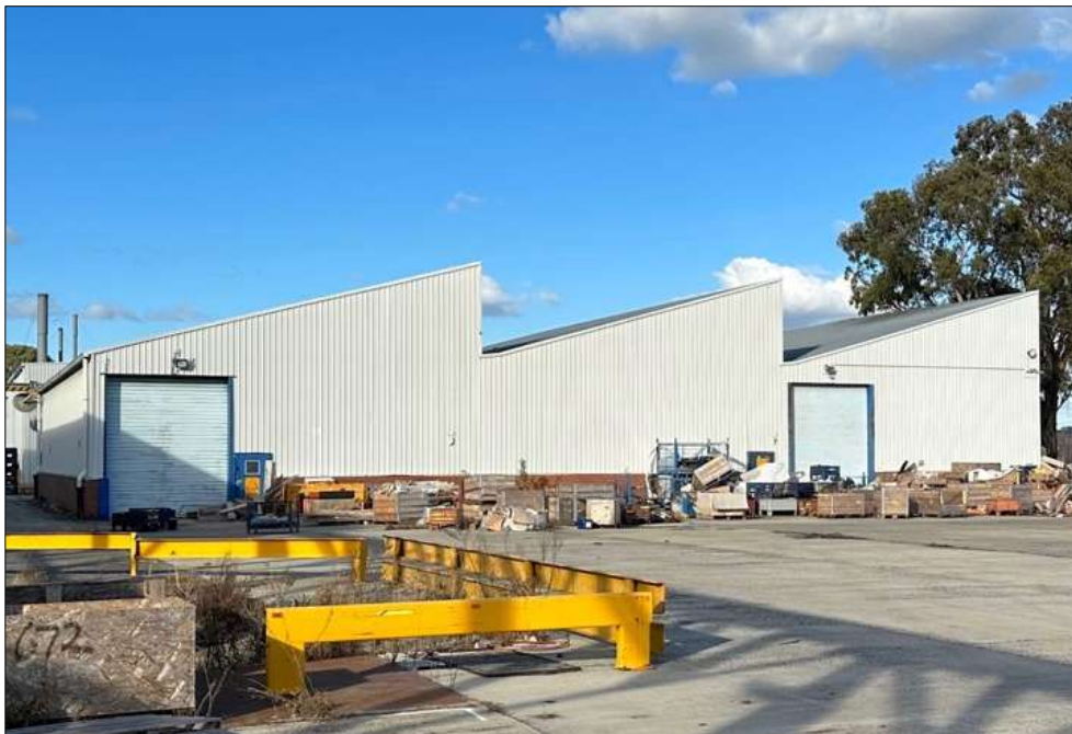
Figure 17 The c1957 sawtooth roof warehouse to the south of the main factory.
