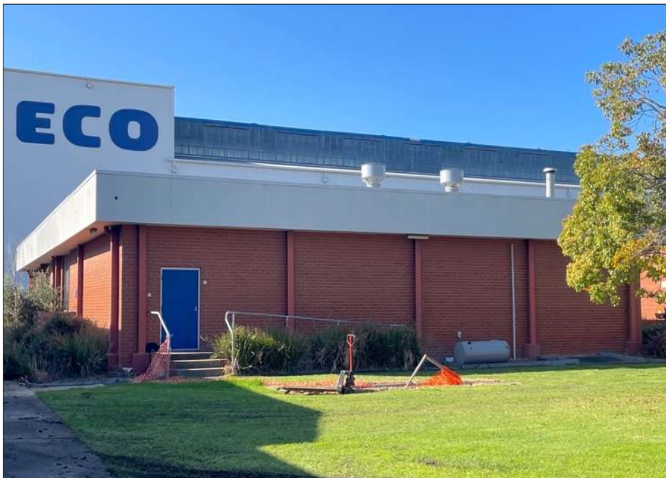
Figure 26 The c1990s building to the rear of the administration building.
