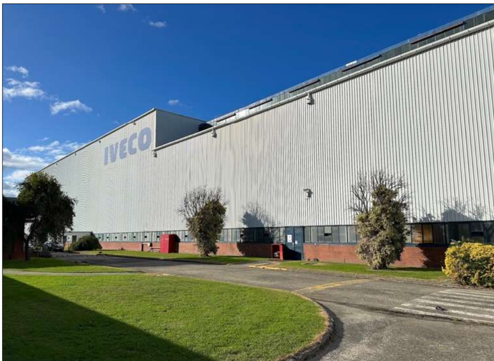
Figure 11 The west elevation of the 1950s crane bay and its c1968-72 addition (left).
