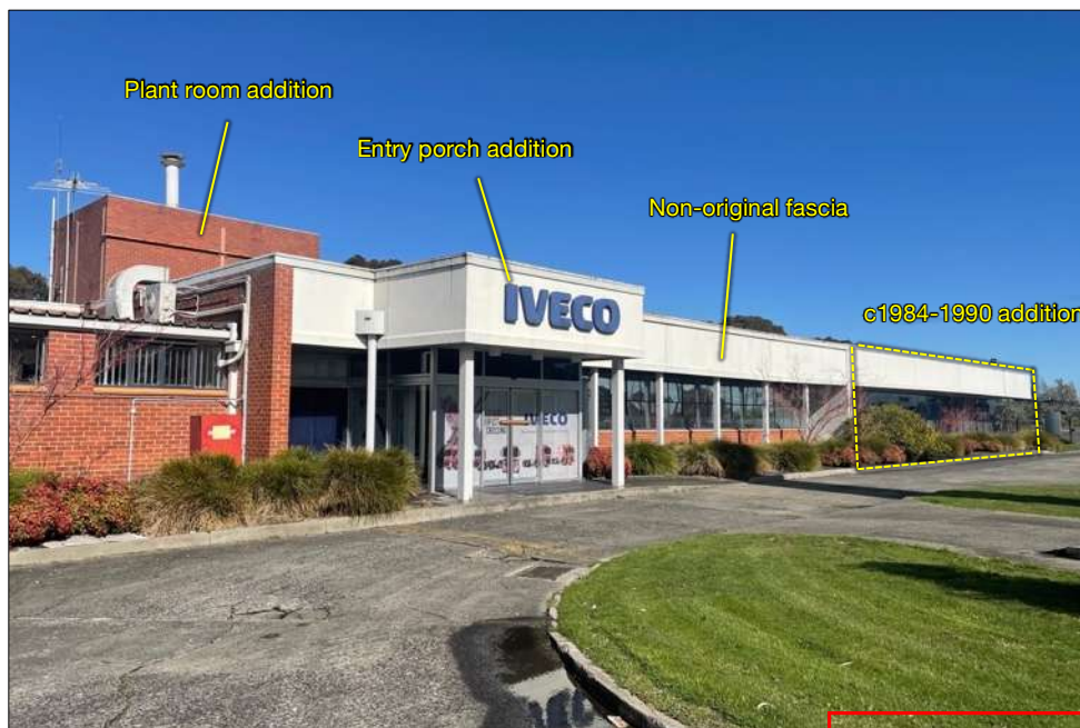
Figure 22 Current view of the administration building's façade.
