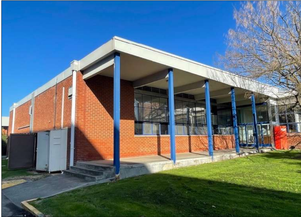
Figure 23 The c1954 addition to the administration building, viewed from the north-east.
