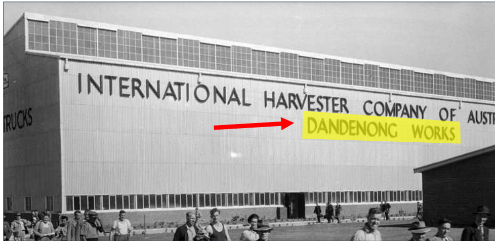
Figure 33 1953 photograph of the crane bay showing the original 'Dandenong Works' signage
