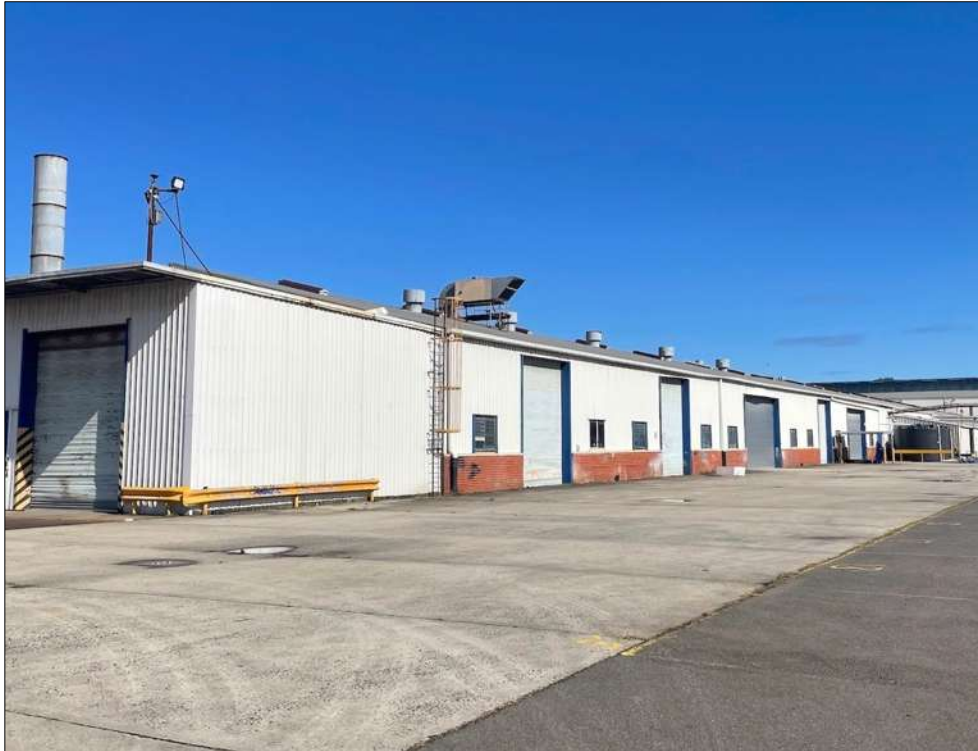
Figure 14 The north elevation of the main factory building.
