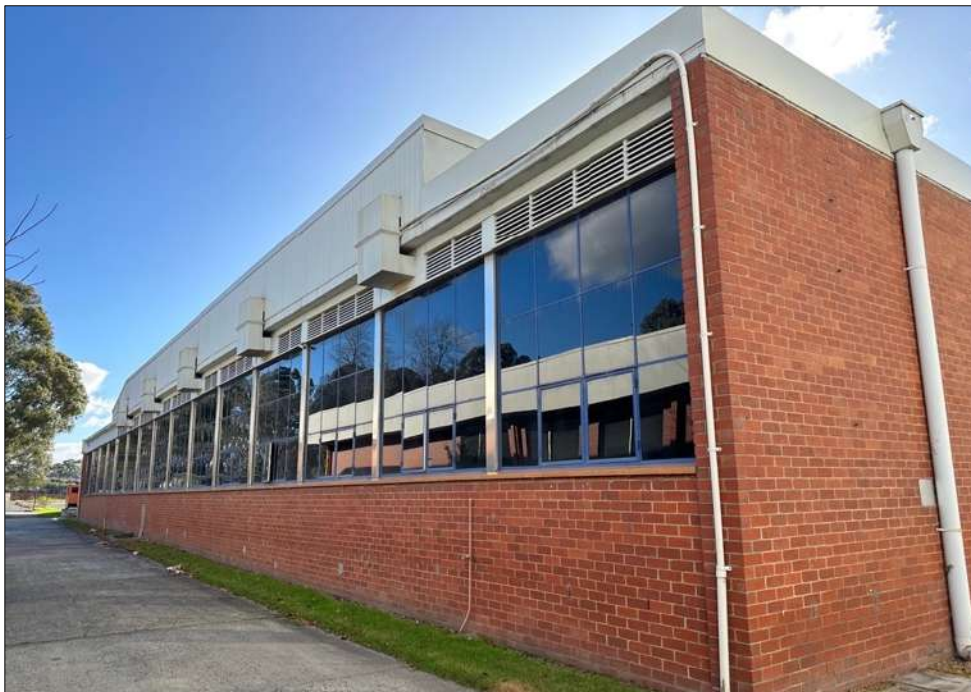
Figure 24 The south elevation of the c1954 addition.
