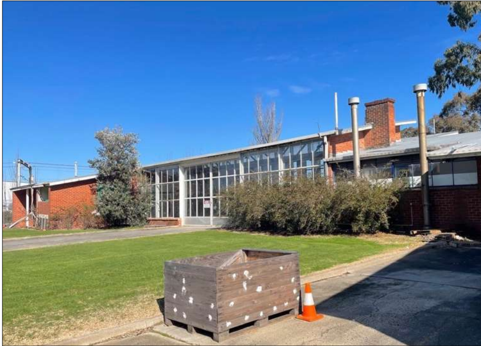
Figure 27 The east elevation of the amenities block.
