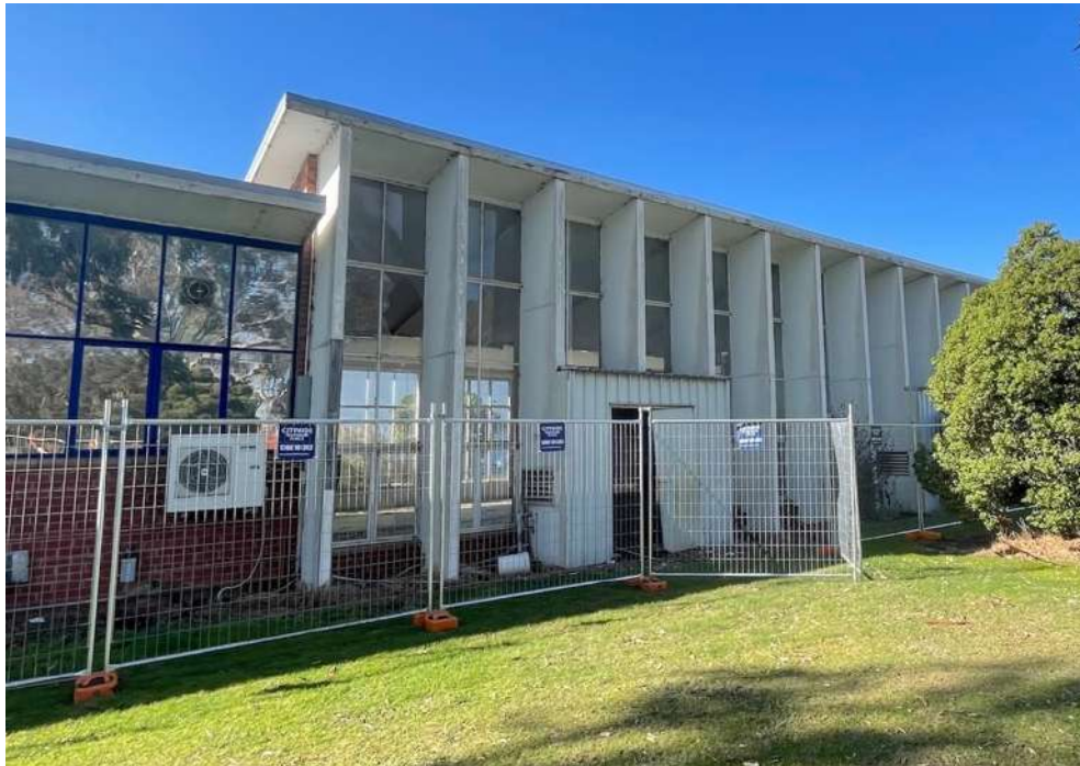
Figure 28 Partial view of the amenities block west elevation showing the vertical sun baffles.
