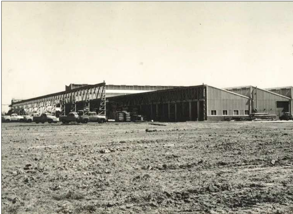
Figure 5 The factory viewed from the south east, c1953. Source: Hassell.
