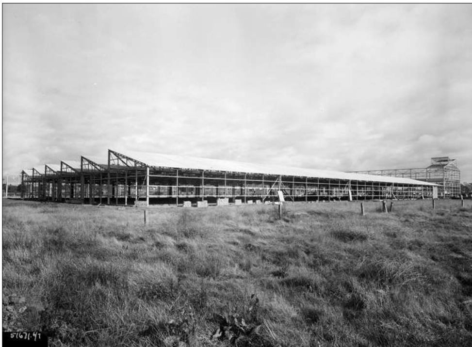
Figure 1 The factory under construction, 1951. Source: Museum Victoria
