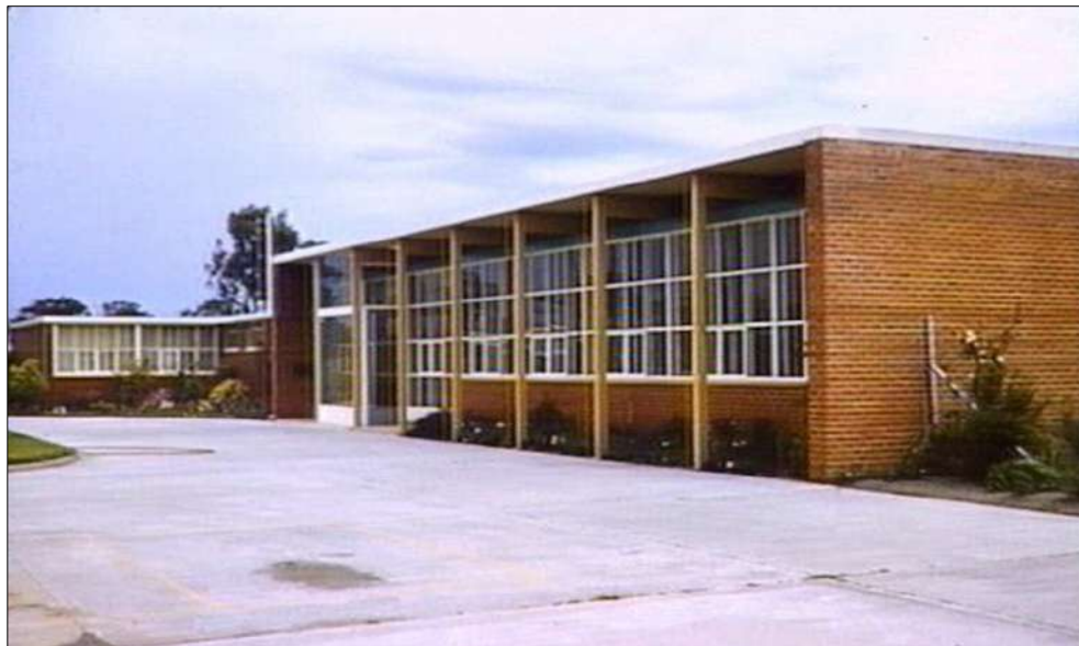
Figure 3 The administration building, 1953. Source: State Library of Victoria.
