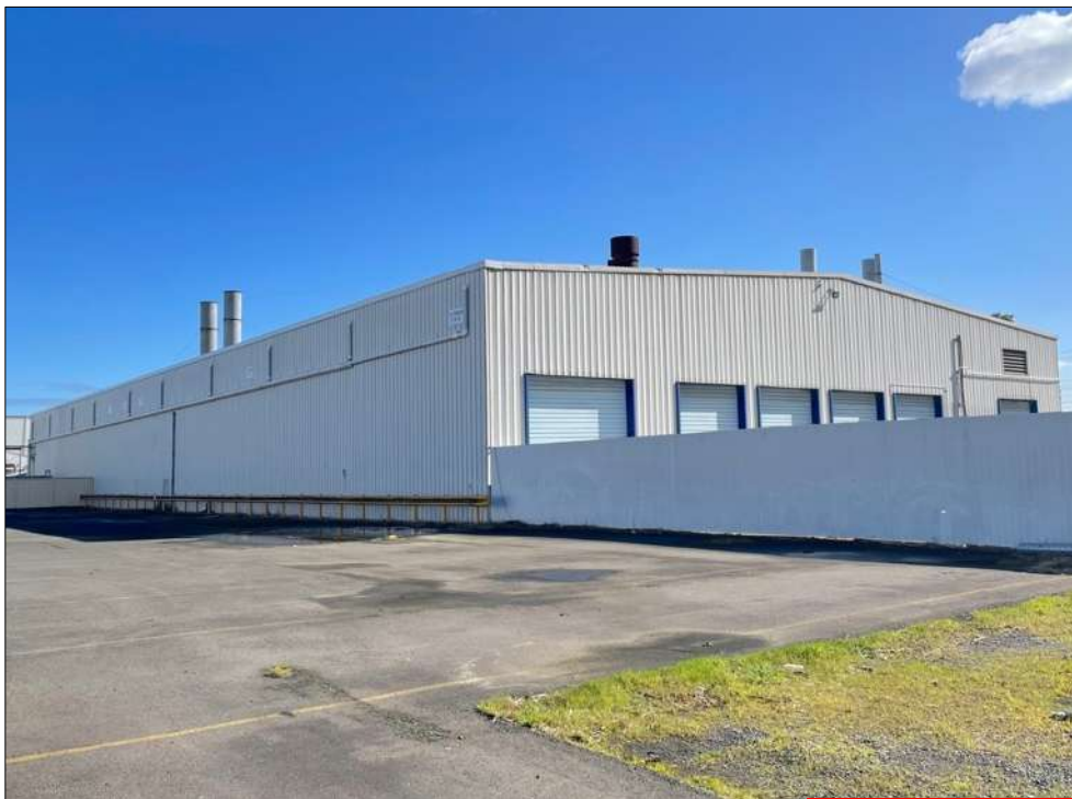
Figure 15 1977 building to the north-east of main factory.
