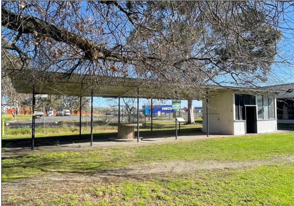
Figure 25 The bicycle shed.
