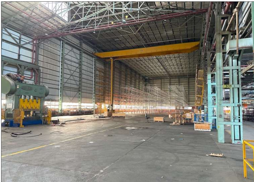
Figure 19 The interior of the crane bay looking north towards the c1968-72 addition.
