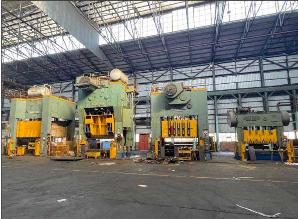
Figure 20 Mechanical presses inside the crane bay.
