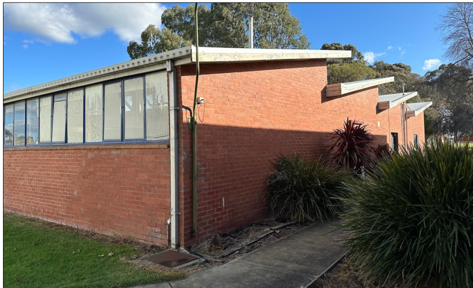
Figure 3 Northern end of the Amenities Building now proposed for retention.
