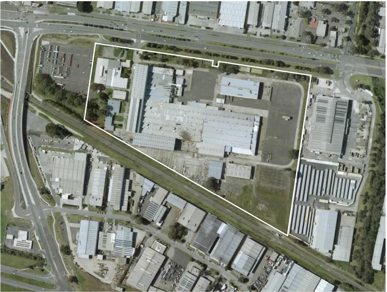
Figure 2: Aerial image of the development site at 7 Princes Hwy, Dandenong South (Source: LandChecker)
