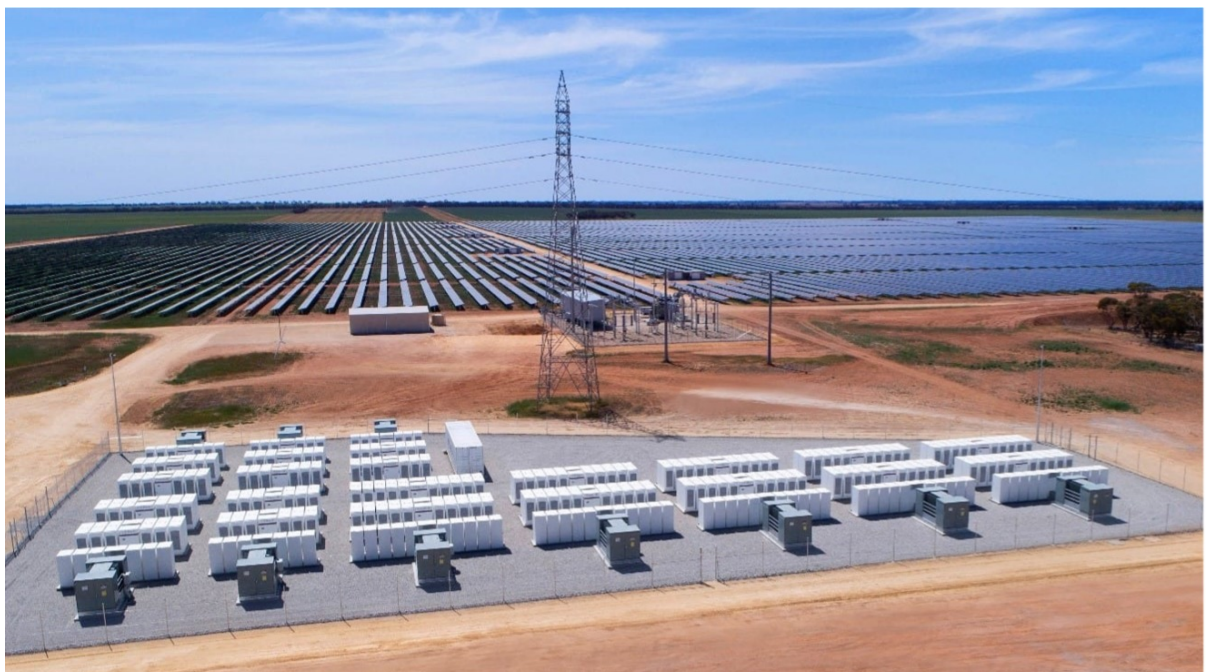
Figure 3 Illustration of a type of BESS coupled with a solar farm (source: www.energyaustralia.com.au/about-us/energy-generation/gannawarra-battery-storage )
