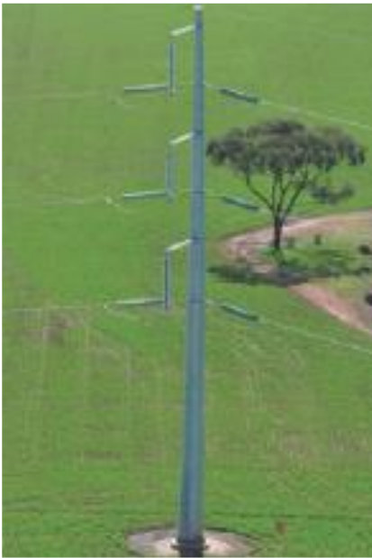
FIGURE 81 – INDICATIVE 220 KV STRAINER POLE CONFIGURATION
