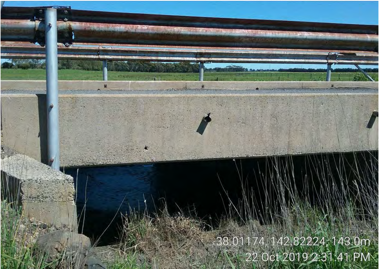
Photo 11 Bridge over Blind Creek on South Road
