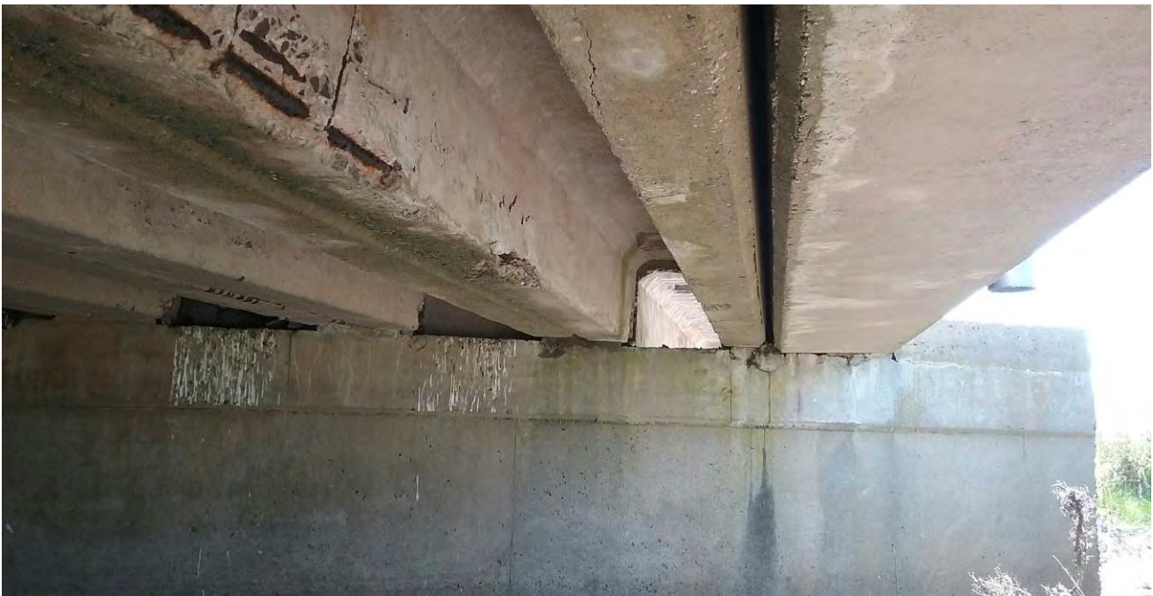
Photo 12 Underside of bridge over Blind Creek on South Road
