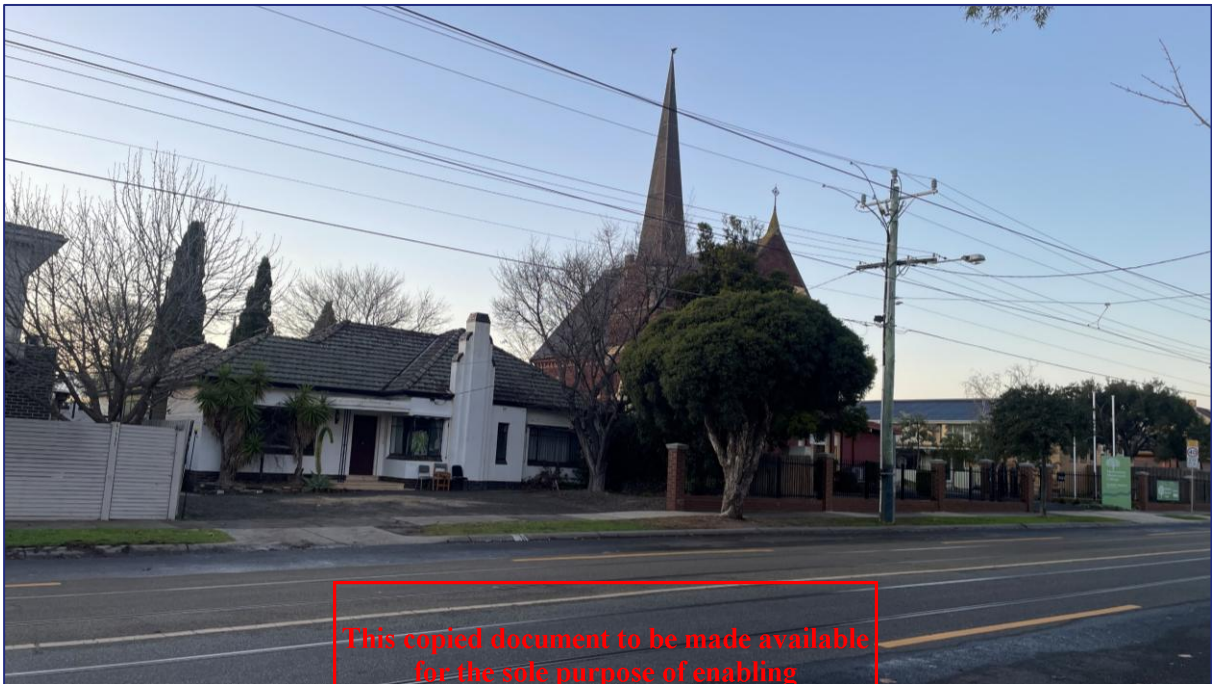
Figure 1: Subject Site (view south-east from Hawthorn Road)
