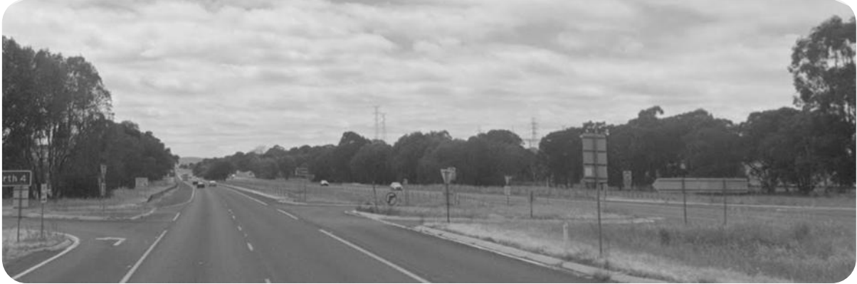
Figure 4 Hume Freeway facing east
