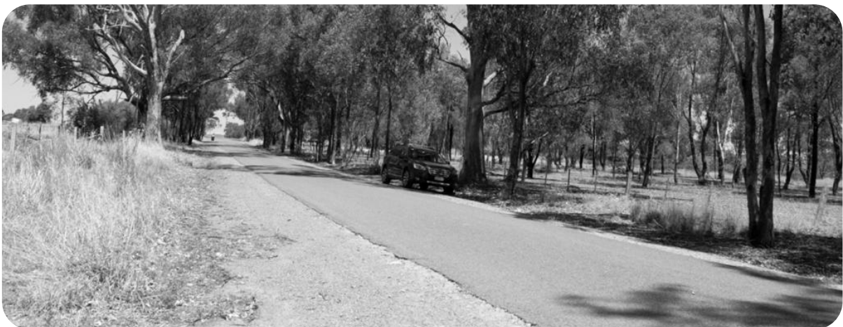
Figure 3 View of Bowers Road facing south adjacent the subject site
