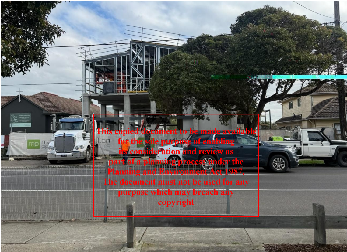
Figure 10: The construction site viewed from the opposite side of Minerva Road.
