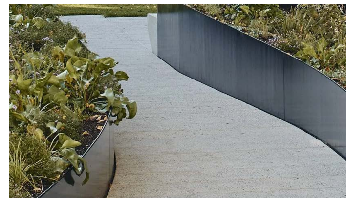
Garden beds are created from black powder-coated steel blade walls, slicing through the organic brick, stone and timber materiality.
