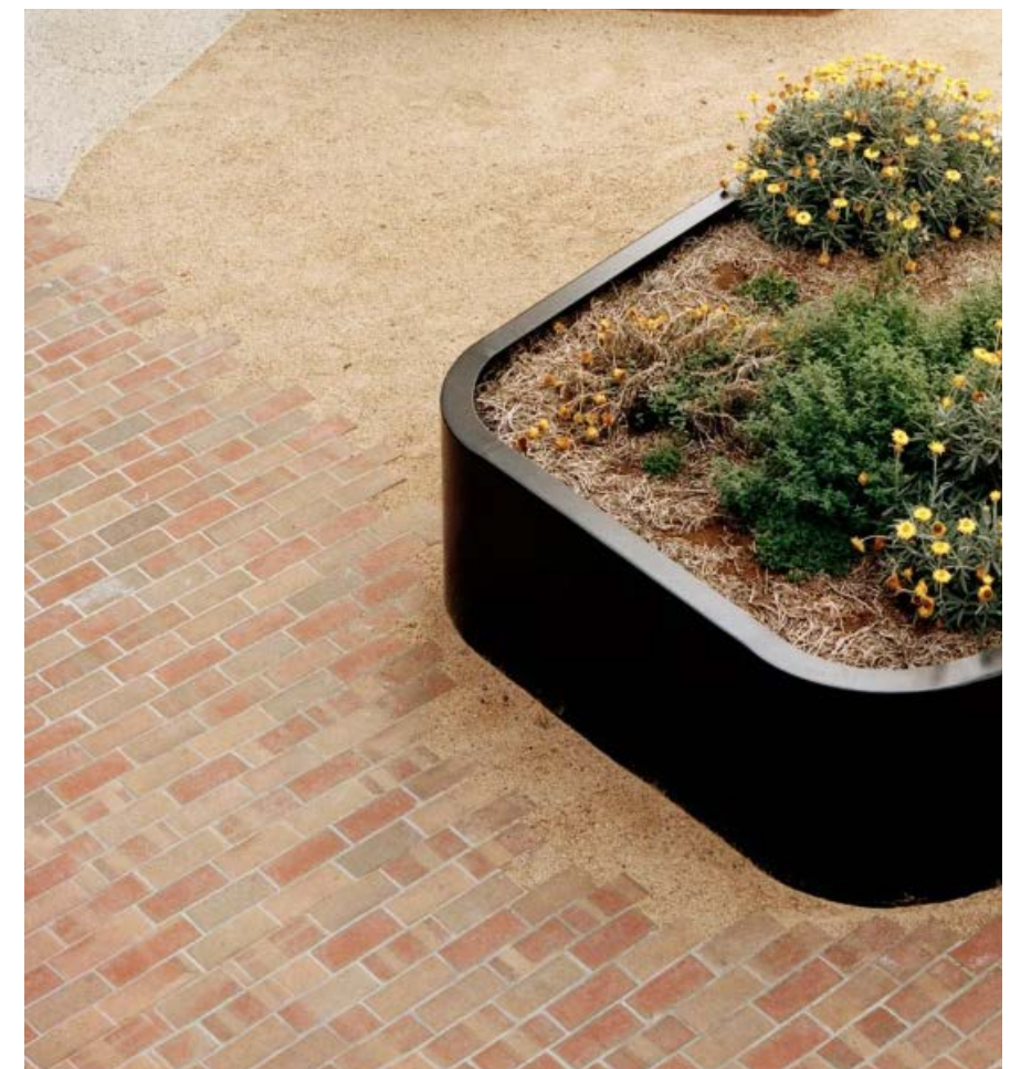
Within the site, black powder-coated steel planters maximise soil volume and planting with a ground plane of multi-coloured brickwork
