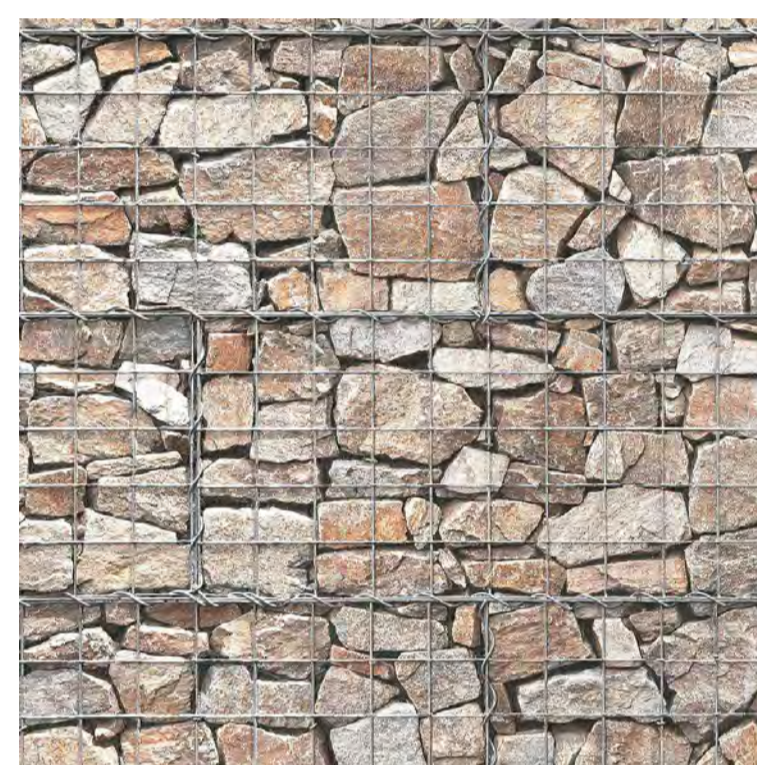
GABION WALL Hornfels Rock Mawsons Quarry (or similar)
