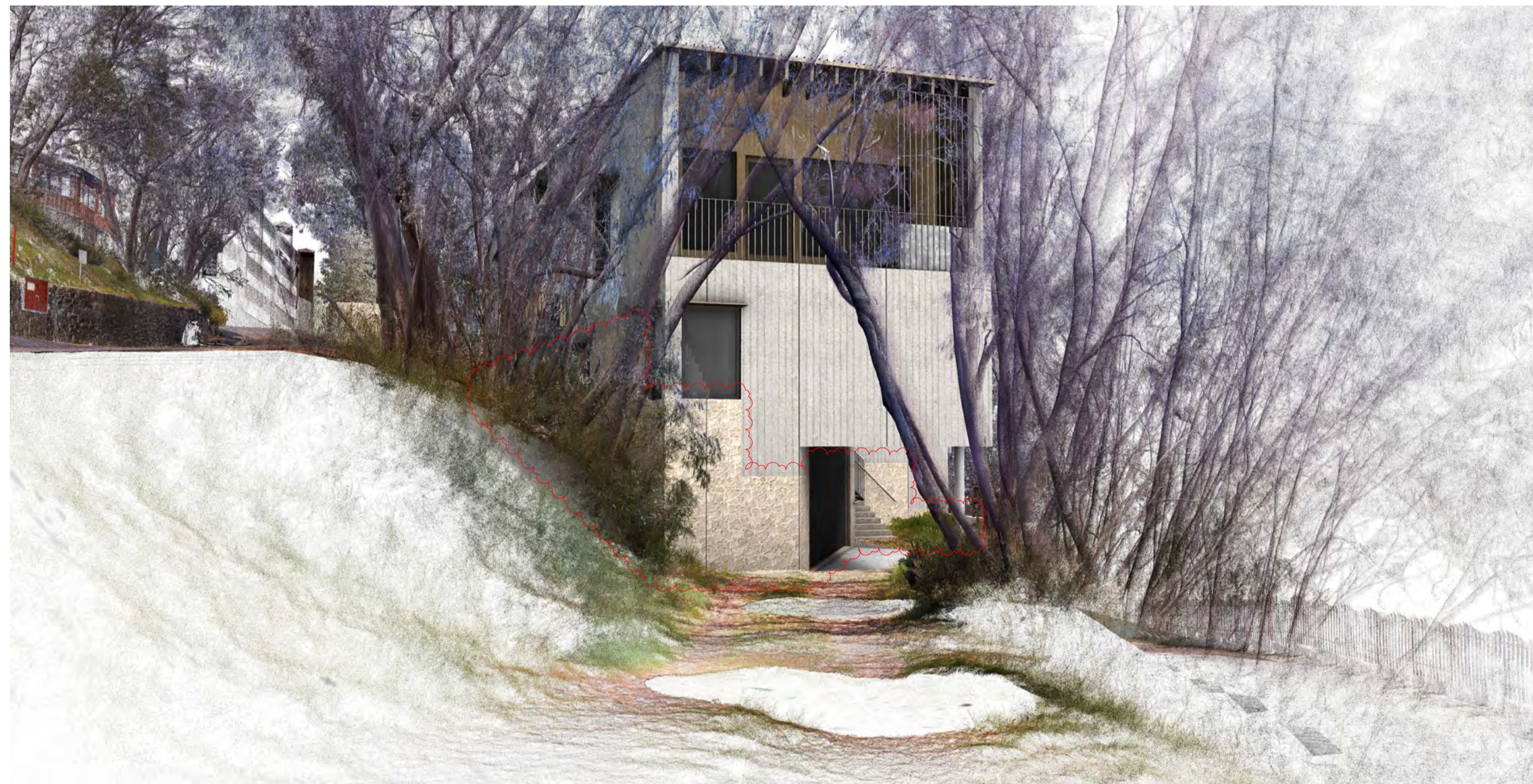
VIEW FROM 'ADJACENT PARCEL' ACCESS PATH LOOKING SOUTHWEST (SUMMER ACCESS)
