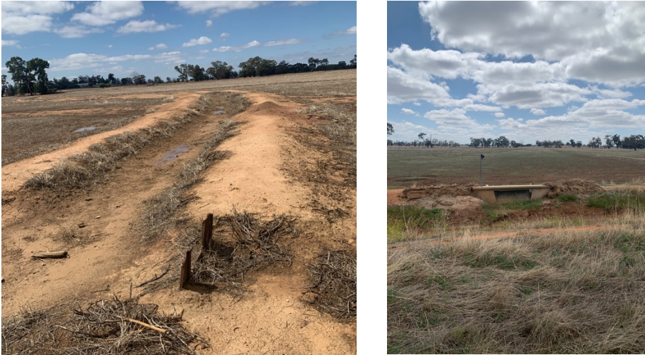
Figure 3-6: Examples of bay outlets on farm channels
