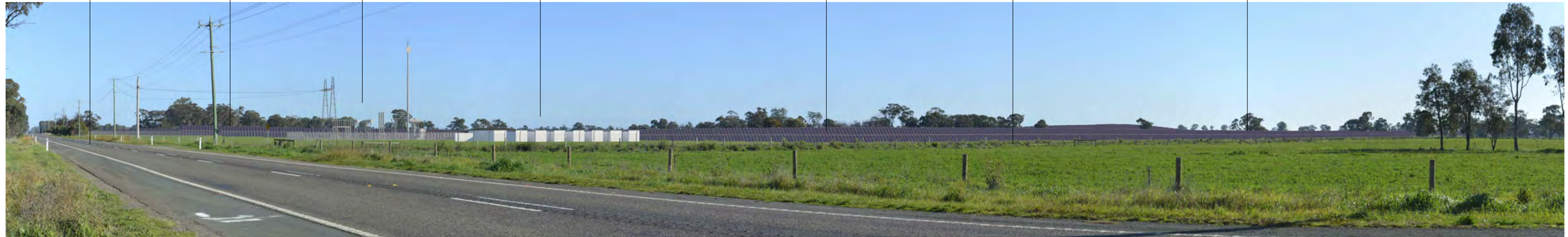
Photomontage PM1 Proposed view post construction toward Viewbank Solar Farm site from Midland Highway
