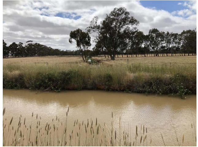
Figure 3-4 Photo 2, on top of the irrigation channel bank facing east
