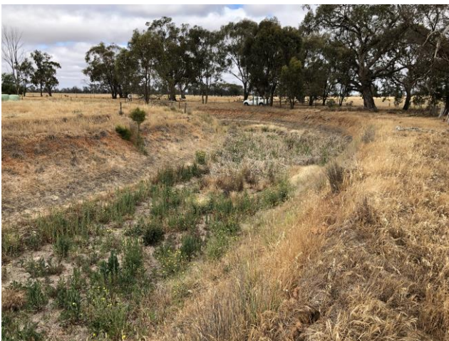
Figure 3-5 Photo 3, irrigation dam, facing west
