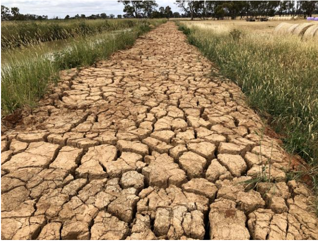
Figure 3-3 Photo 1, on top of the irrigation channel bank facing south
