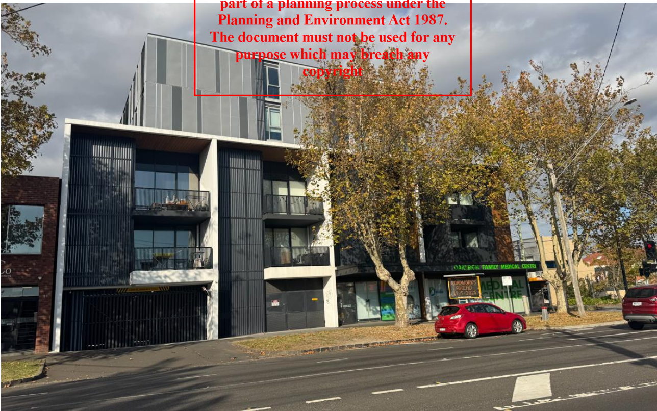
Figure 16 – Eastern interface of the subject site – 63-65 Atherton Road (apartment development with commercial component) (photo taken May 2025)
