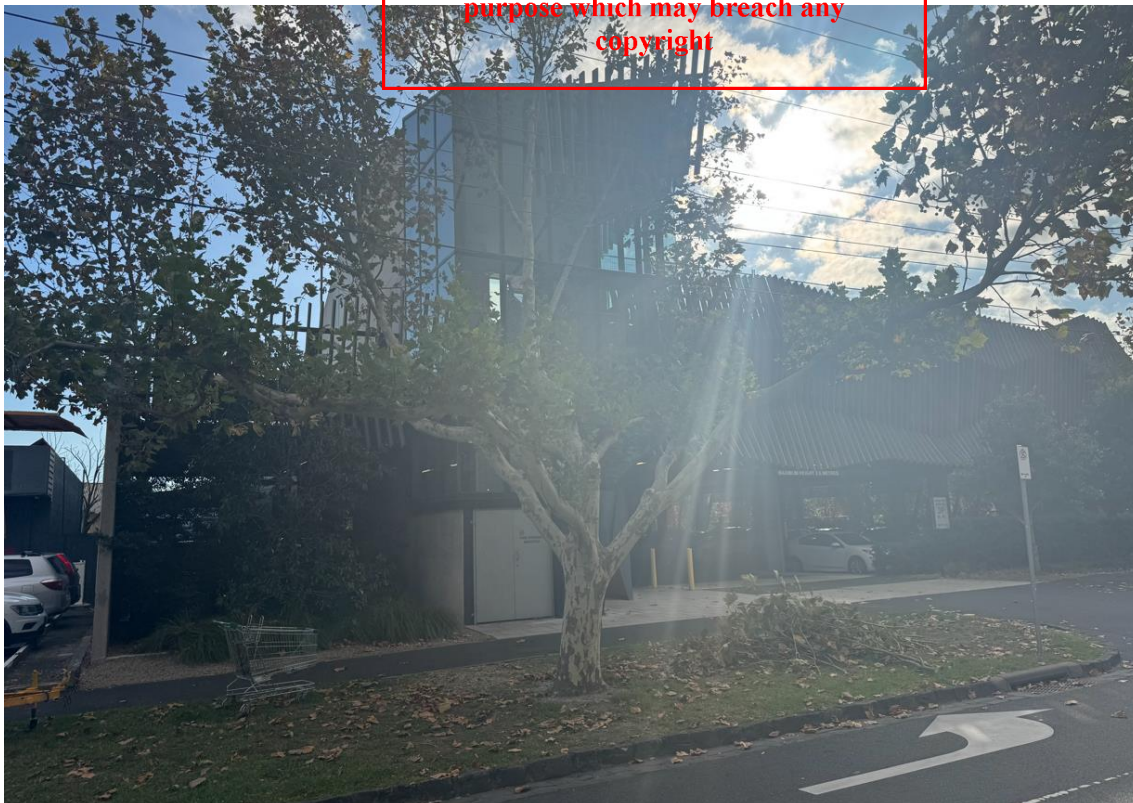
Figure 14 – Northern interface of the subject site – 129-133 Atkinson Street (Atkinson St carpark)
