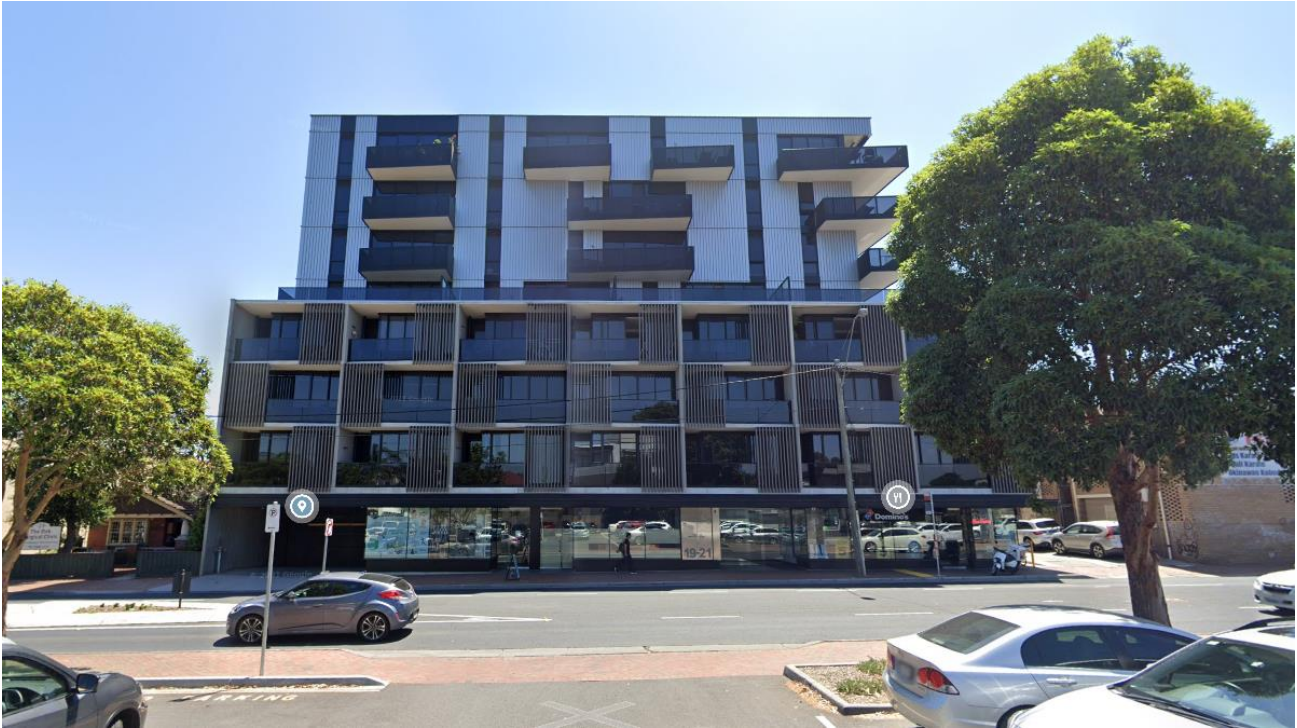
Figure 21 – 19-21 Hanover Street – street view (google maps, January 2019)
