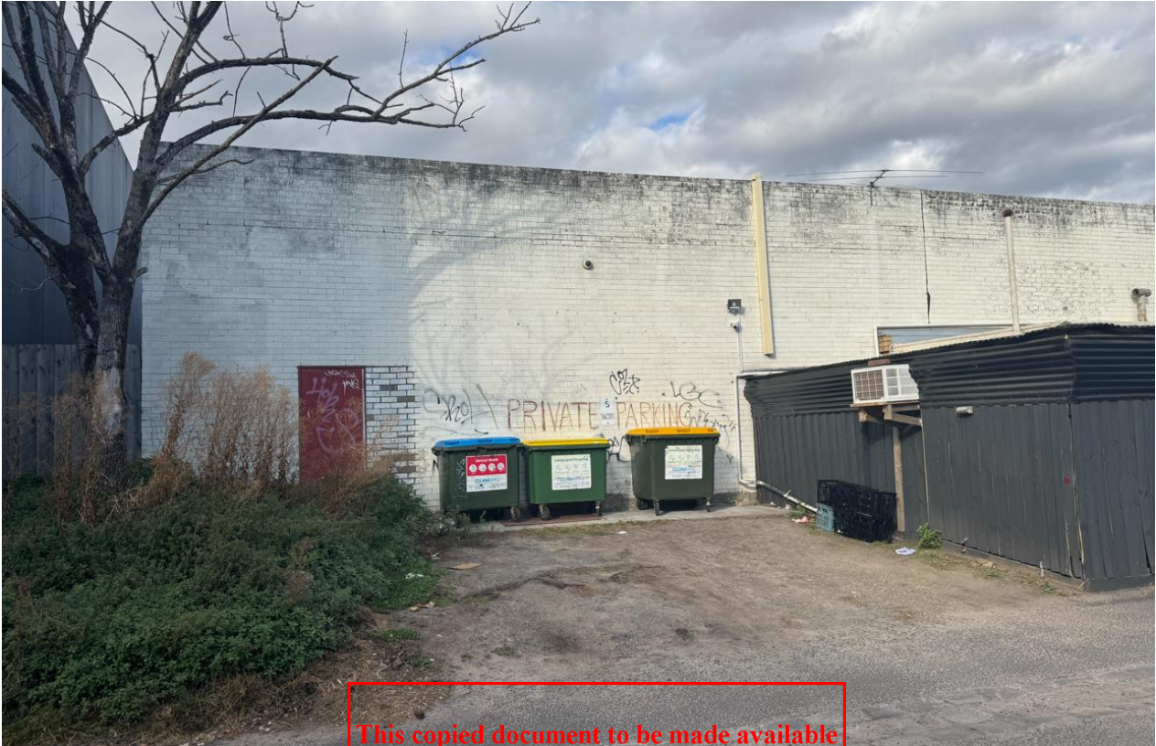
Figure 12 – Subject site – view from western side laneway (photo taken May 2025)
