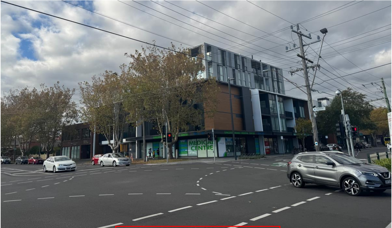
Figure 19 – View of 63-65 Atherton Road – mixed-use apartment development (photo taken May 2025)
