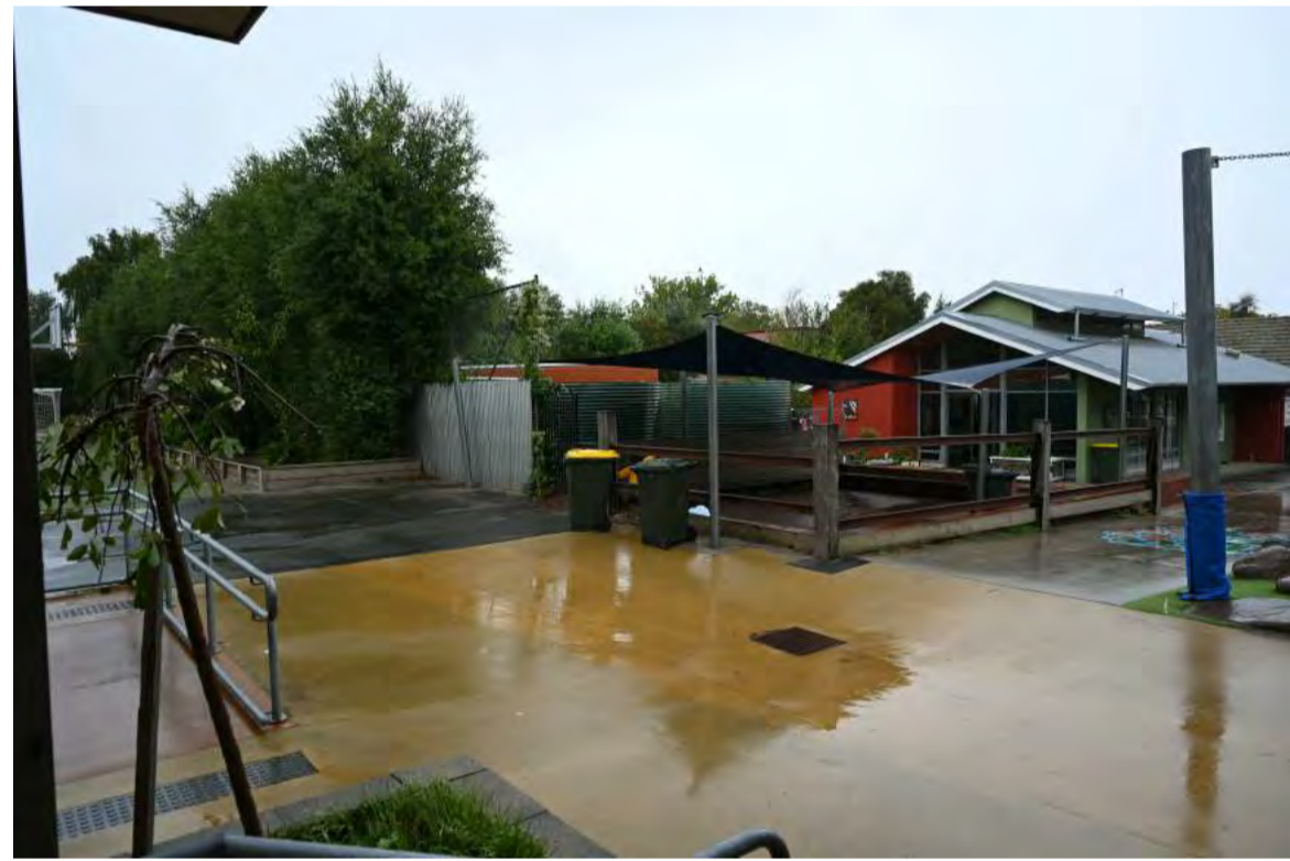
11- VIEW FROM MAIN BUILDING TOWARD ENVRIO SCIENCE BUILDING
