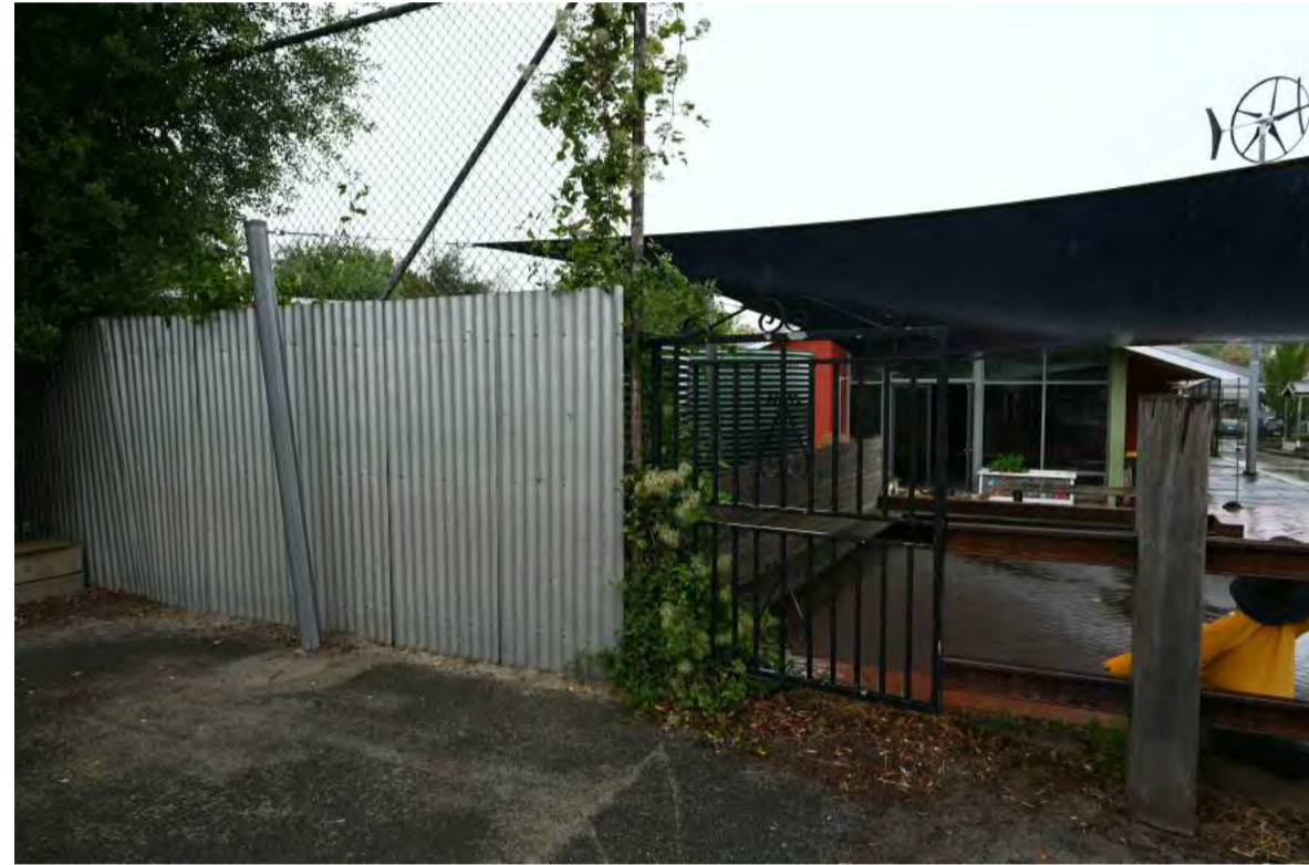
9- VIEW OF MULTIPURPOSE BUILDING SITE
