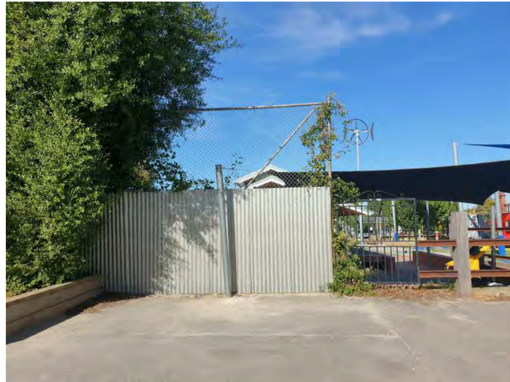
8- EXISTING CORRUGATED AND CHAIN WIRE BOUNDARY FENCE
