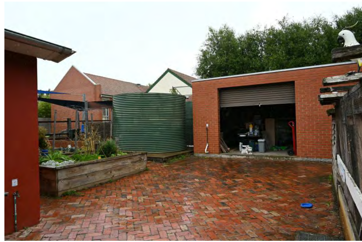
18- EXISTING SHED AND RAIN WATER TANKS
