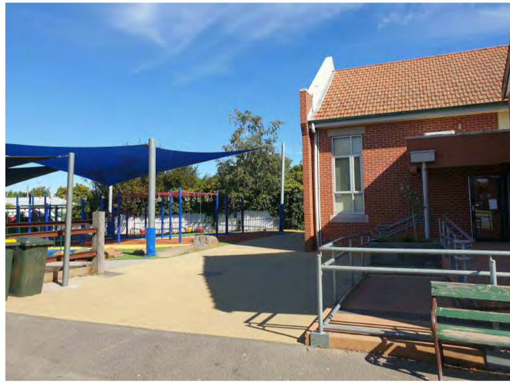
12- VIEW OF MAIN BUILDING AND PLAYGROUND
