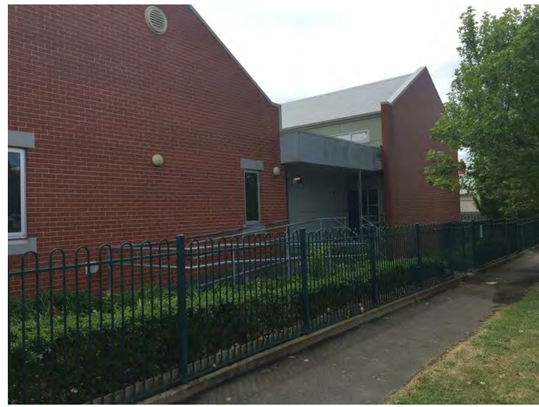
5- STREET VIEW FROM EYRE ST
