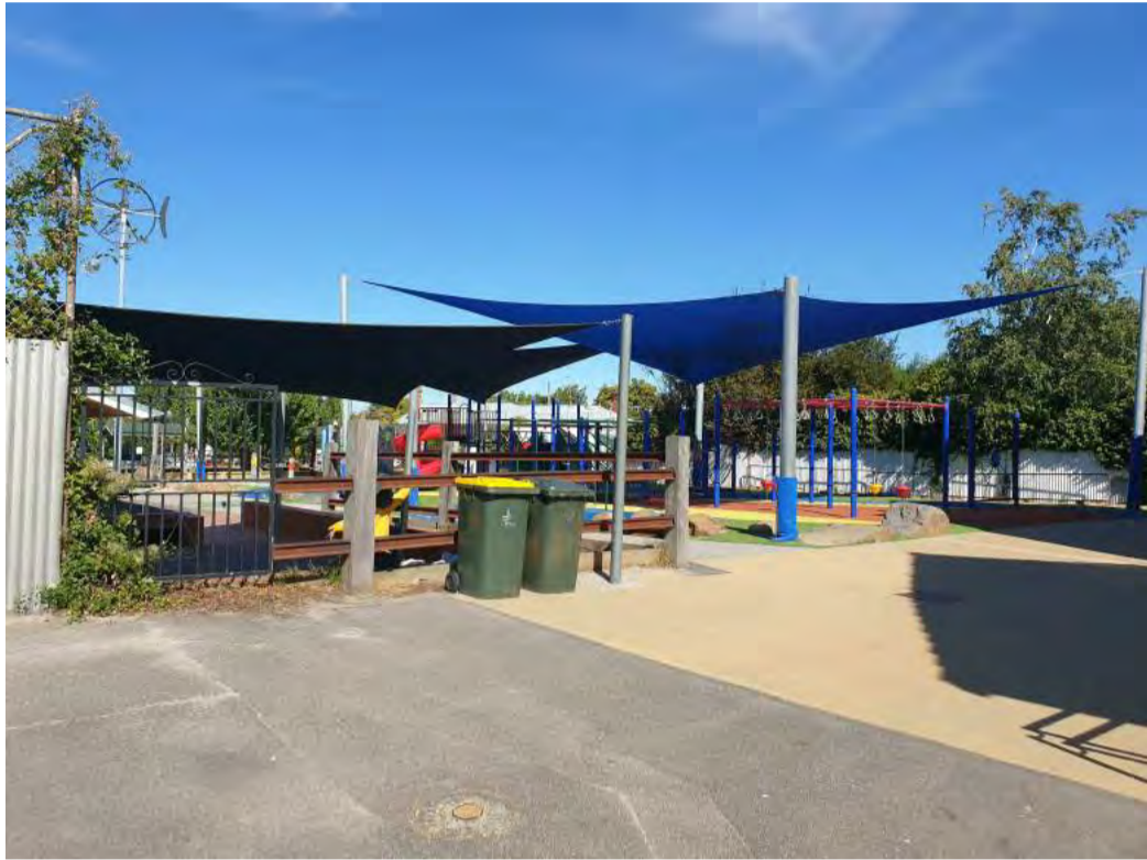
10- VIEW OF MULTIPURPOSE BUILDING SITE AND PLAYGROUND BEYOND
