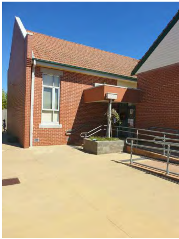
14- VIEW OF MAIN BUILDING PLAYGROUND ENTRY AND STAIRS/RAMP
