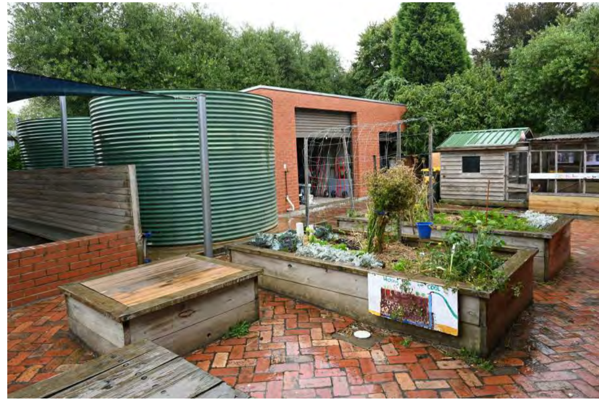
19- SEWER MAIN ACCESS ENCLOSURE, GARDEN BEDS AND CHICKEN COOP
