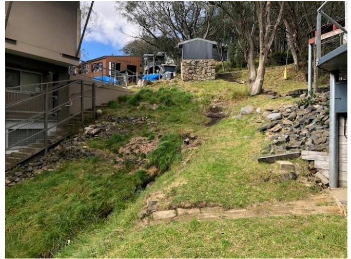
Site Photo 2: Walkway surrounding area
