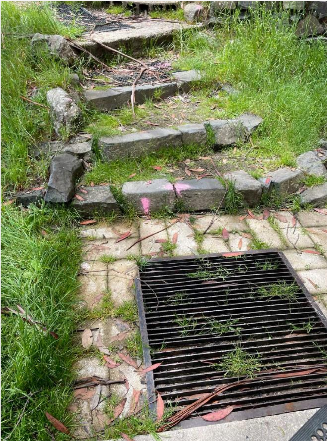
Figure 4 | Existing Conditions of the Current Walkway
