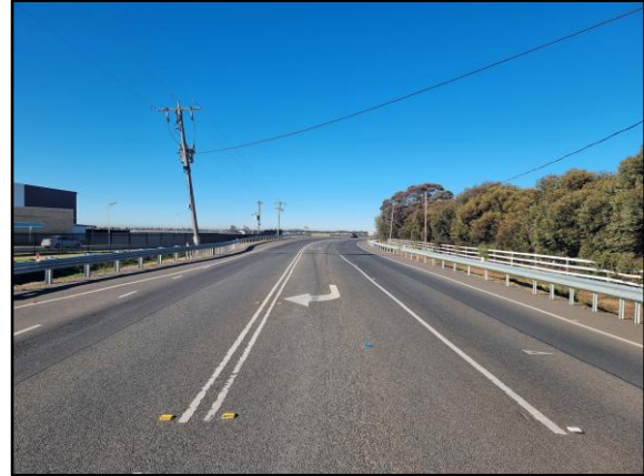
Figure 5: Coburns Road - View South
