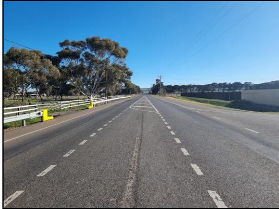
Figure 4: Coburns Road - View North
