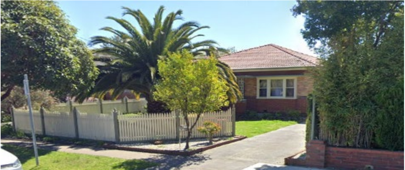
Picture 7: 13 King Street, Dandenong (looking north-west)
