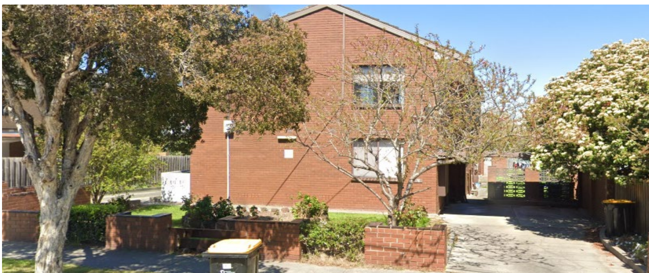
Picture 4: No. 4 Edith Street, Dandenong (looking south)
