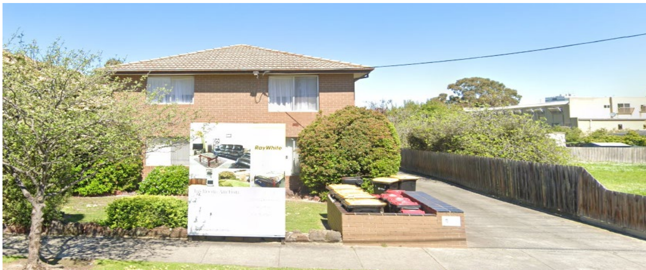
Picture 3: No. 2 Edith Street, Dandenong (looking south)
