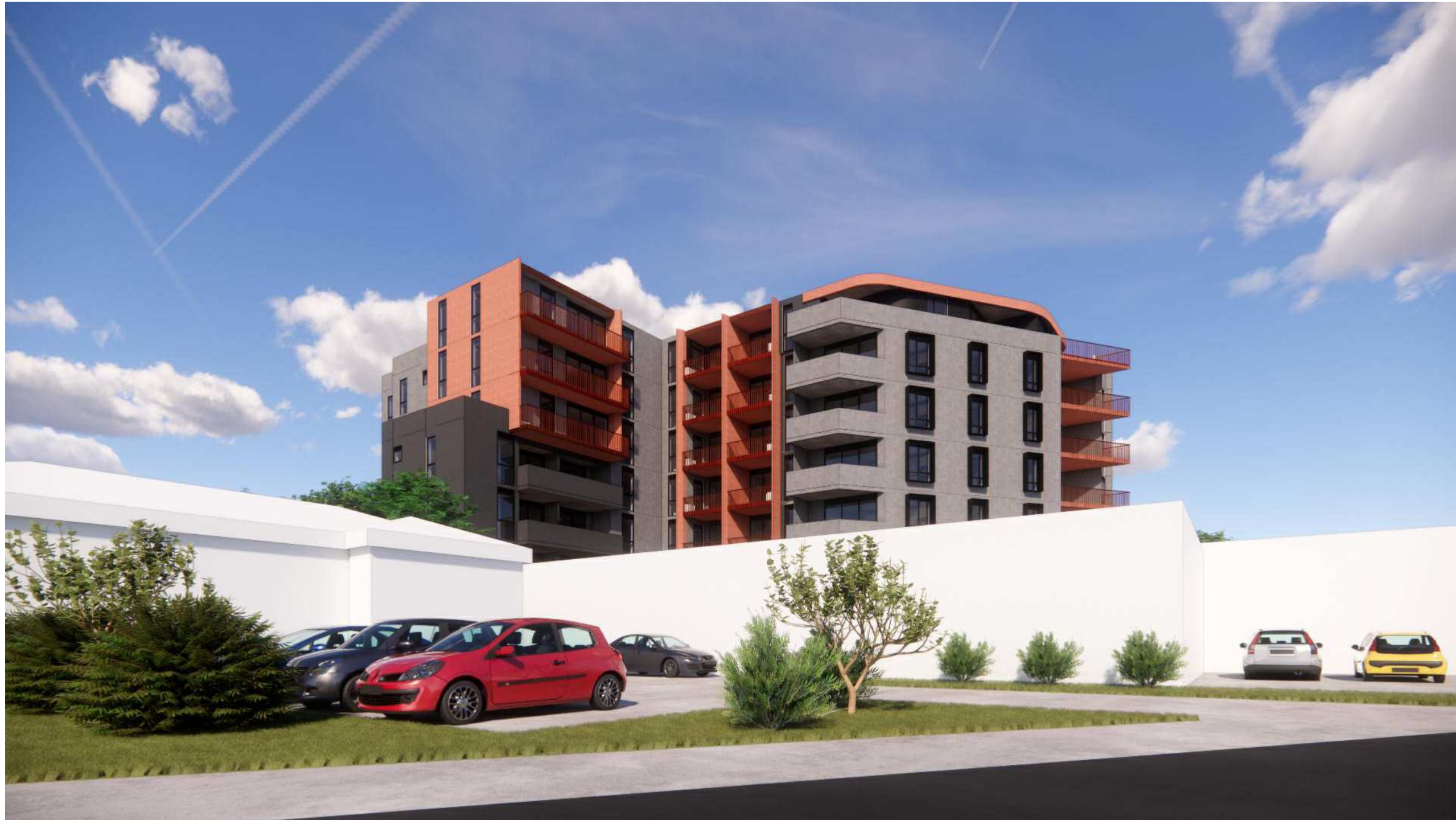
VIEW 04 - NORHTERN & EASTERN FACADES VIEWED FROM LIGHTWOOD RD
